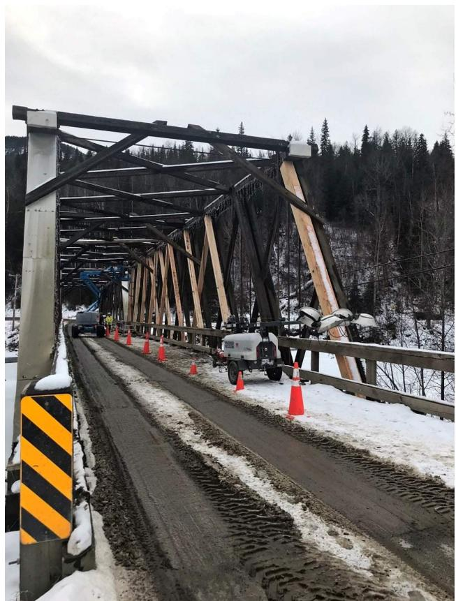
Figure 15 Ongoing Diagonal Replacement Work
