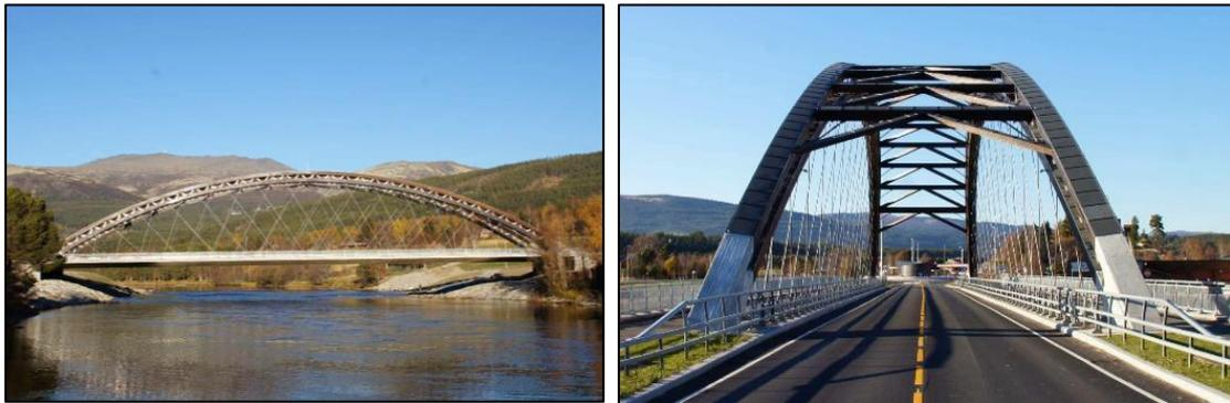
Figure 3. Photo of the structural principle of the bridge (bridge) and out-of-plane stabilization (right) [9]
