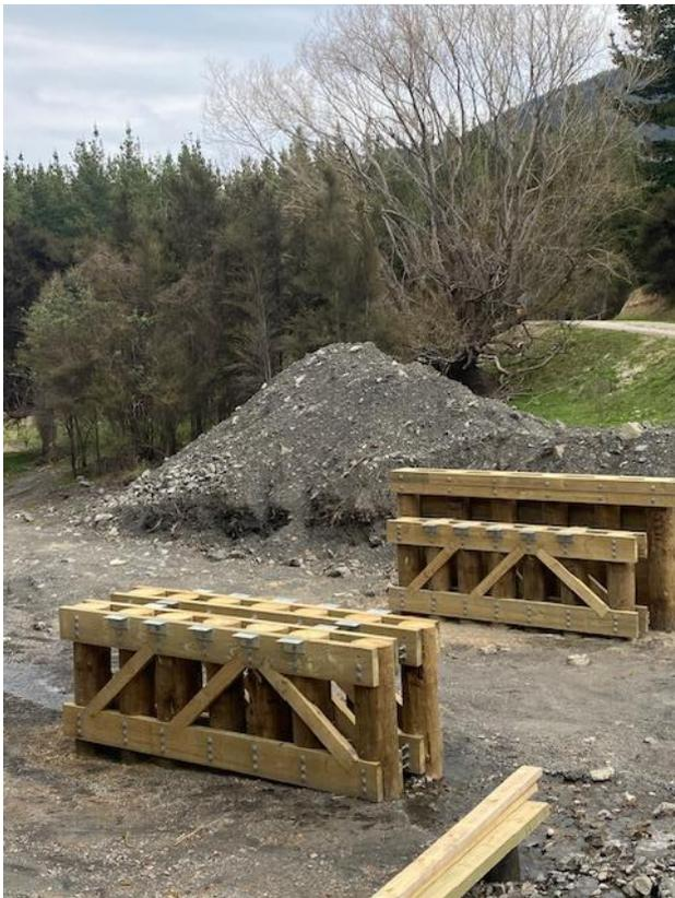
Photo 8: Abutment and mid-span support structure.
