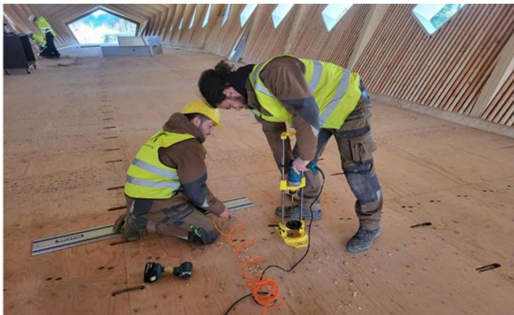
Figure 7: Drilling the holes for the wood moisture measuring points
