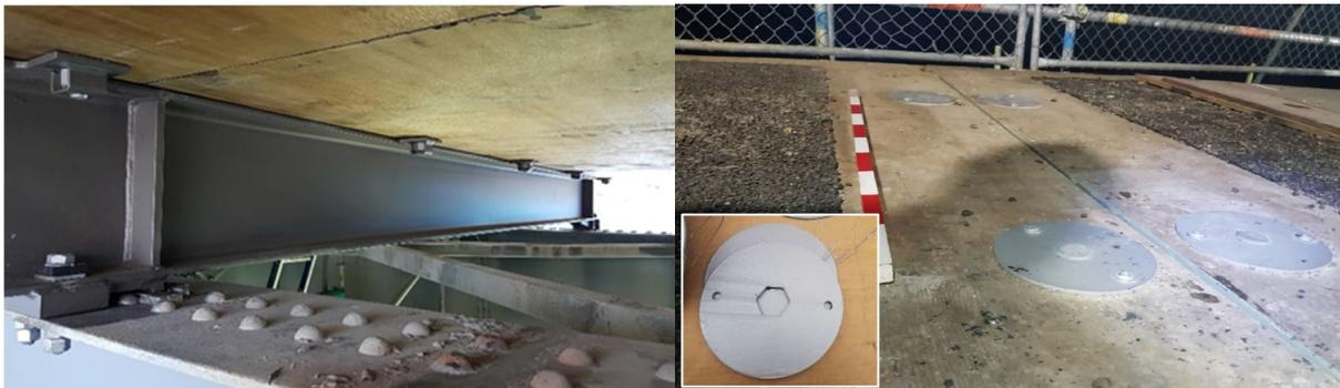
Figure 11. Transom and deck panel connections.
