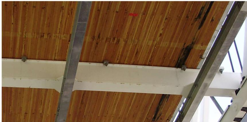
Figure 5. SLT deck and cross girder support
