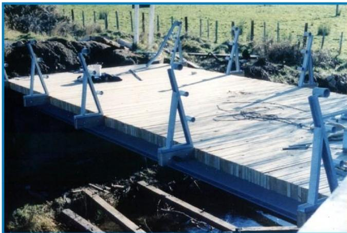
Figure 1(a). Longitudinally post-tensioned timber deck supported on steel beams.
