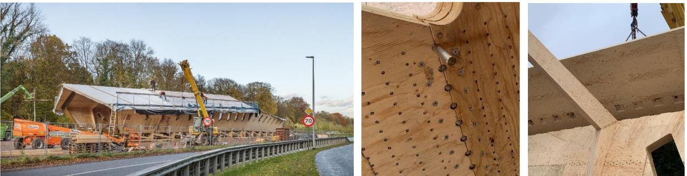
Figure 12. Assembly of GLVL panels on the prefabrication area ©Ney & Partners
