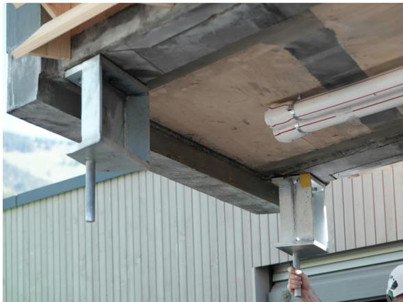
Figure 29: Detail of the fixed support and service lines
