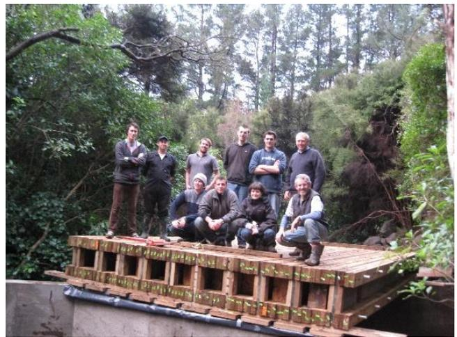
Figure 3. The timber bridge after construction in one day, before tensioning.
