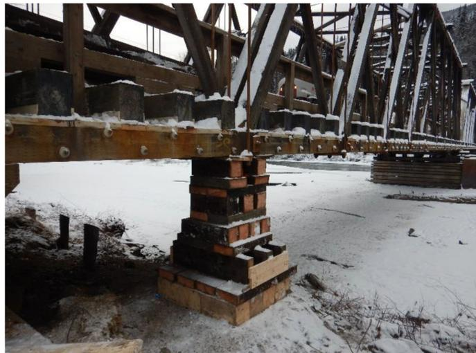
Figure 11. Temporary Shoring Installed Under Panel Point
