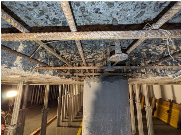
Figure 9: Strengthening of a ceiling using UHPFRC, Reichenburg, Switzerland
