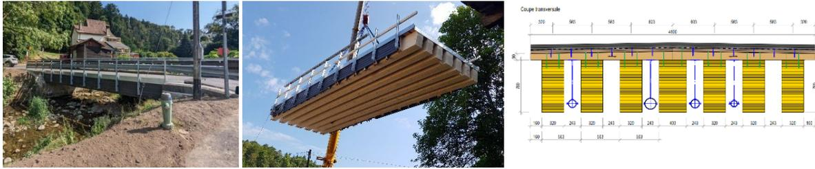
Figure 5. Le Tirage bridge, side view, lifting of bridge deck element, cross section, source: Timbatec Holzbauingenieure Schweiz AG.
