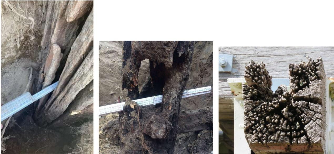
Figure 1: Examples of defects observed in the field in timber pile and beam elements.
