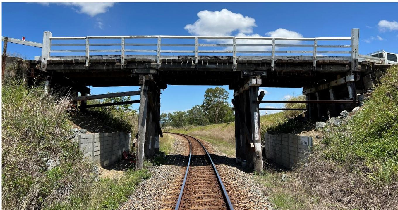
Figure 1. Timber rail overbridge at Hopes Road
