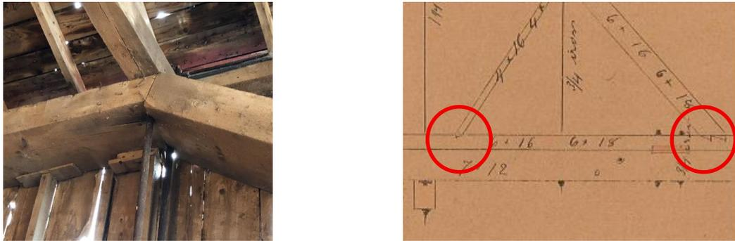
Figure 5. Typical truss node bearing connection (left) and typical truss node notched connection (right).
