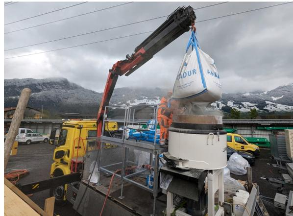
Figure 24: Mixing the UHPFRC on site
