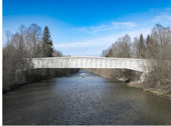
Figure 8: Repair of a historic bridge using UHPFRC, Lauperswil, Switzerland
