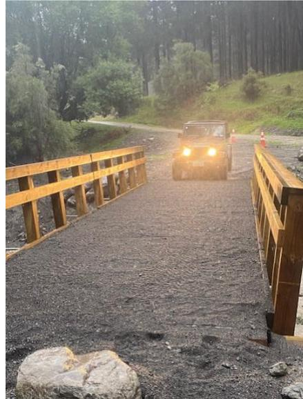
Photo 15: Timber lattice wearing course after application of the gravel surface.
