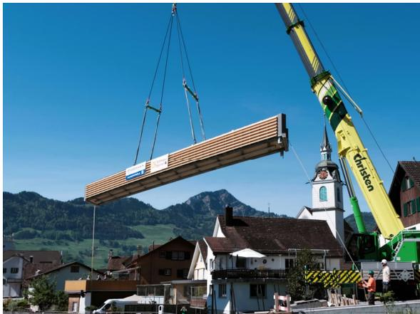
Figure 31: Moving the bridge with a mobile crane
