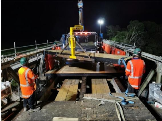
Figure 4 Installation of engineered plywood panels for a recent deck replacement project
