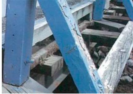
Figure 3. Example bridge section after long term UV radiation [14]
