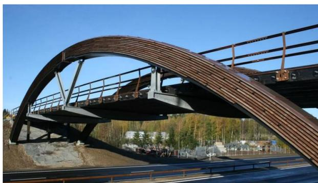
Figure 1. Pinned arch timber bridge in Norway
