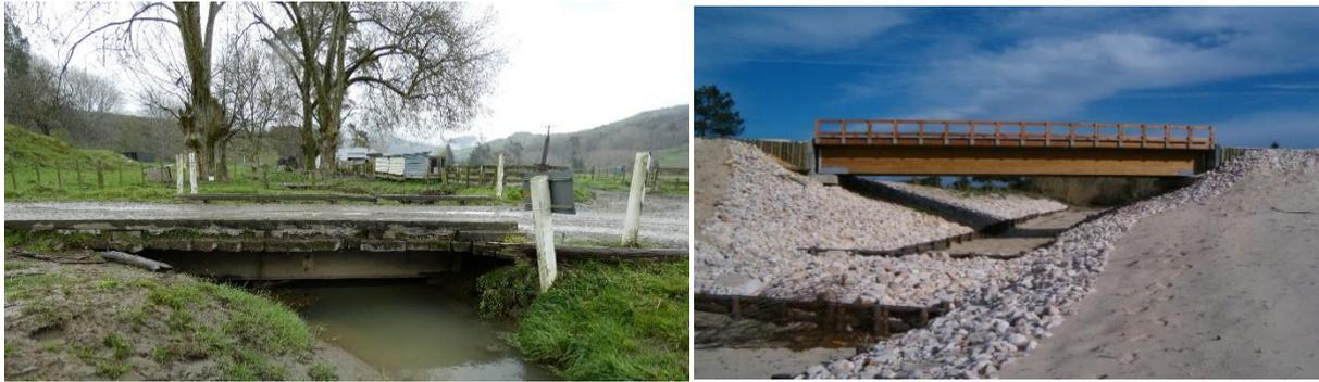
Figure 1. Left, typical New Zealand steel girder bridge with timber deck, Tukemokihi Bridge in Hawkes Bay. Right, timber concrete composite Quiaios Bridge, Portugal [4].
