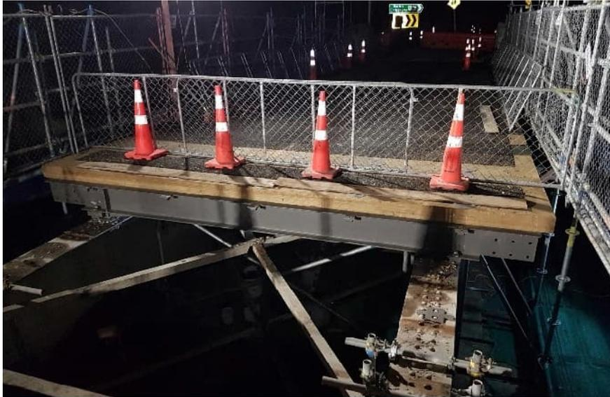
Figure 14. Deck partially removed and replaced.
