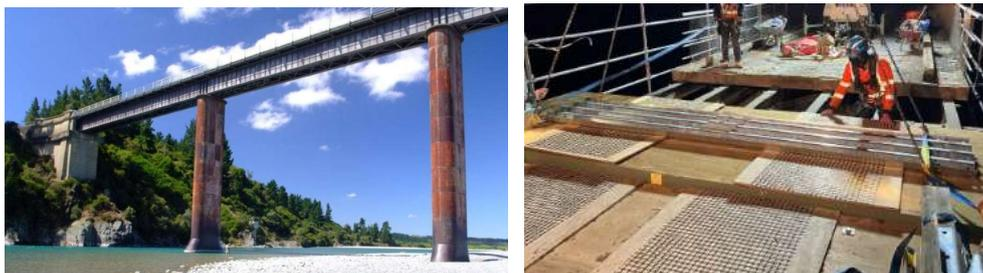
Figure 2. Waimakariri Gorge Bridge (a) Side view [15]. (b) Decking replacement 2024 [16].
