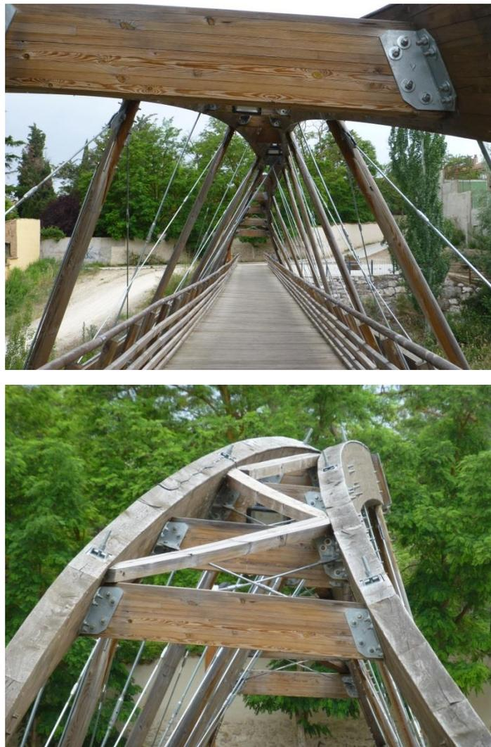
Figures 23 and 24. Failure mode due to buckling.
