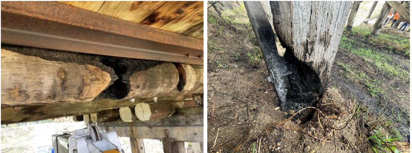
Figure 6. Fire damage (Mid Span Girder left, Pile right) at Wallangarra Rail Overbridge
