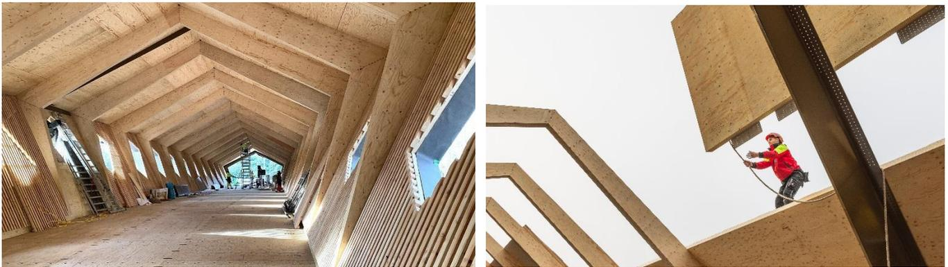
Figure 3. GLVL panel installation
