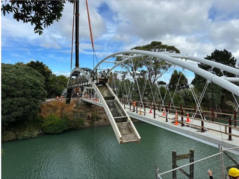
Figure 10. The replacement of the Panmure Basin timber Bridge (March 2025) with a steel structure.
