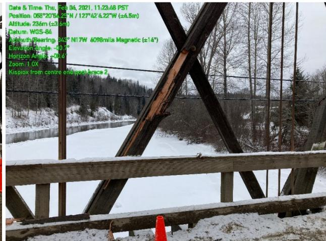
Figure 6. Inner Diagonal With Lesser Damage
