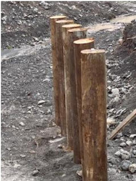
Photo 10: Abutment retaining wall driven timber piles.
