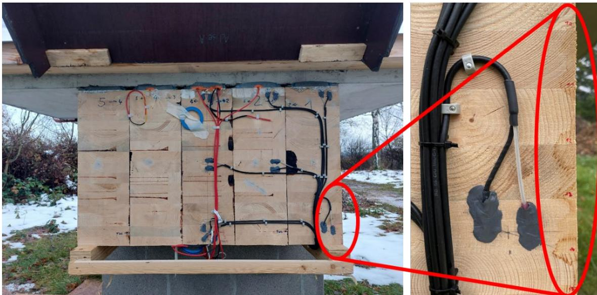
Figure 9. left: North-facing, unsealed end grain of the superstructure segment; right: Water marks close to measuring point FBH-8
