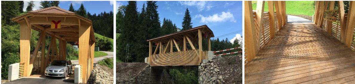
Figure 6. Wühribach bridge, views and flooring with oak planks, source: Timbatec Holzbauingenieure Schweiz AG
