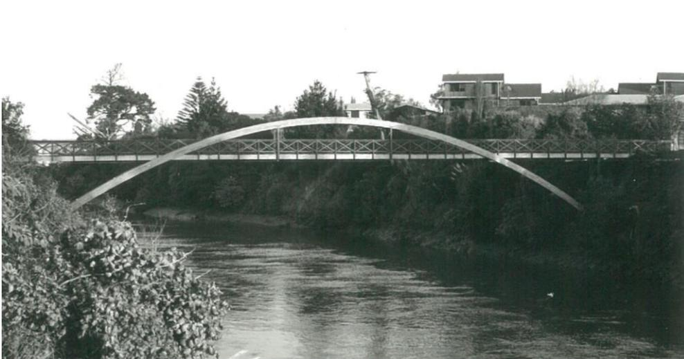
Figure 2 - Panmure basin footbridge, a 60 m long, CCA treated pine structure installed in 1984. Once site works and foundations were in place the wooden bridge structure was completed within a week.
