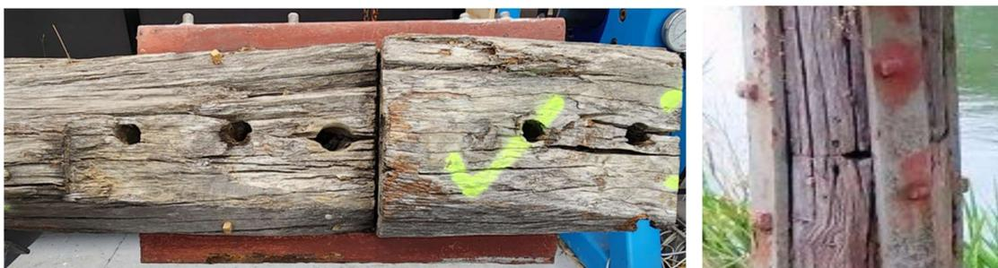
Figure 2: [Left] Historic stump repair on a pile segment removed from service. [Right] Stump repair in service.
