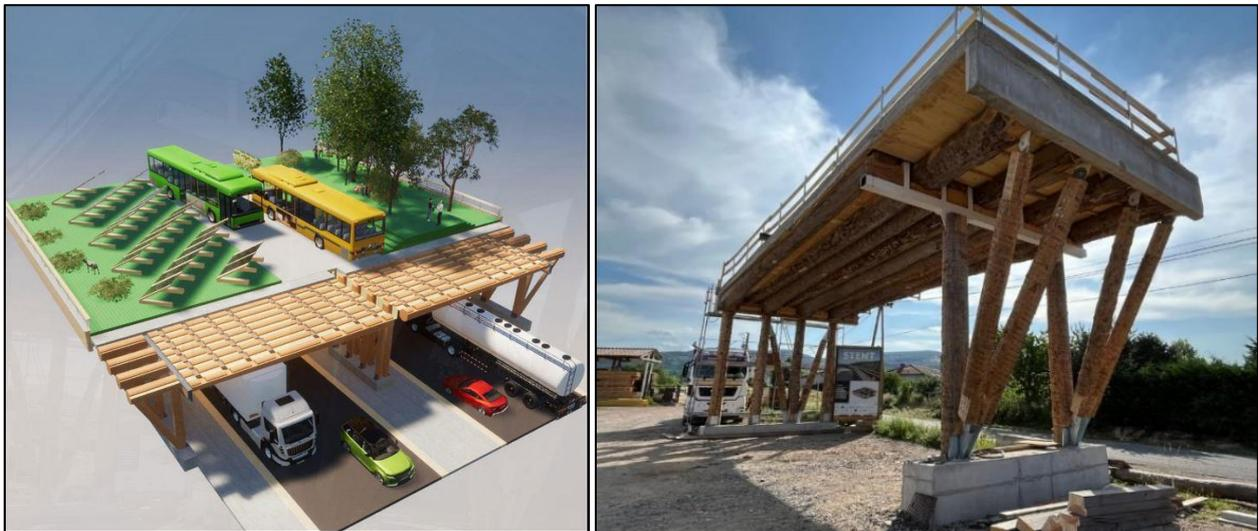
Figure 8. Covering of a highway with a whole log timber crossing structure(left) and Prof of concept of the crossing structure made of a composite concrete-log timber structure (right). (STENT project: <https://www.archipente.com/stent-bois/>)
