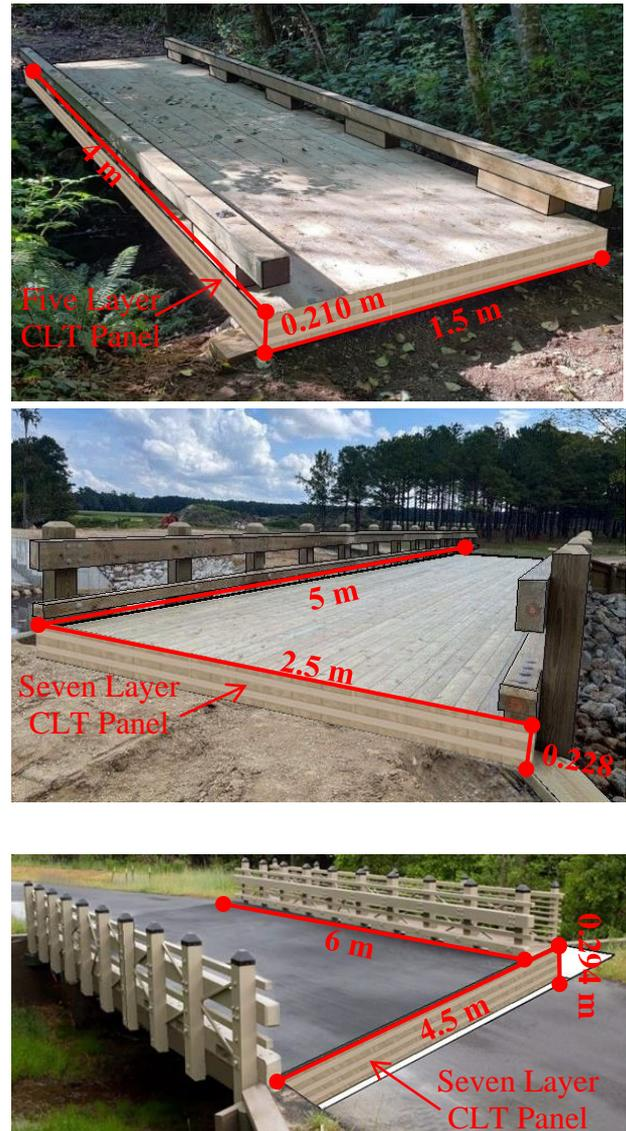
Figure 2. CLT panel application for short-span bridges.
