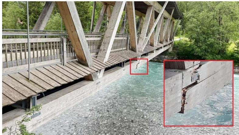
Figure 2. Klimm-Bridge, tension failure at the lower chord [9]
