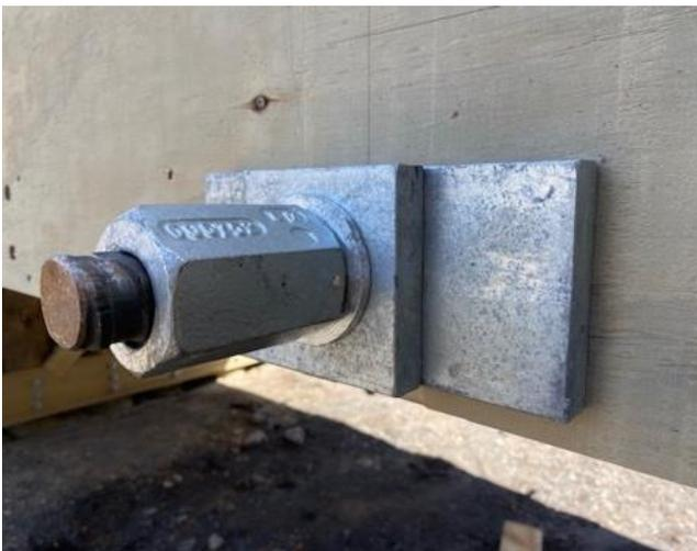
Photo 6: Stress laminated bridge deck stressing bar and bearing plate assembly.
