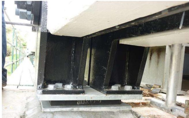
Figure 4. Truss bearings
