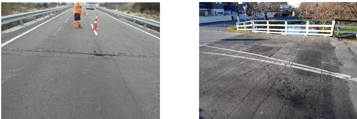
**Figure 5: Surfacing distress on a timber deck state highway bridge (left) and suburban road bridge (right).**
