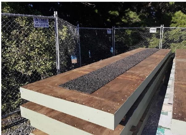
Figure 5. NiuDeck panels ready for installation.
