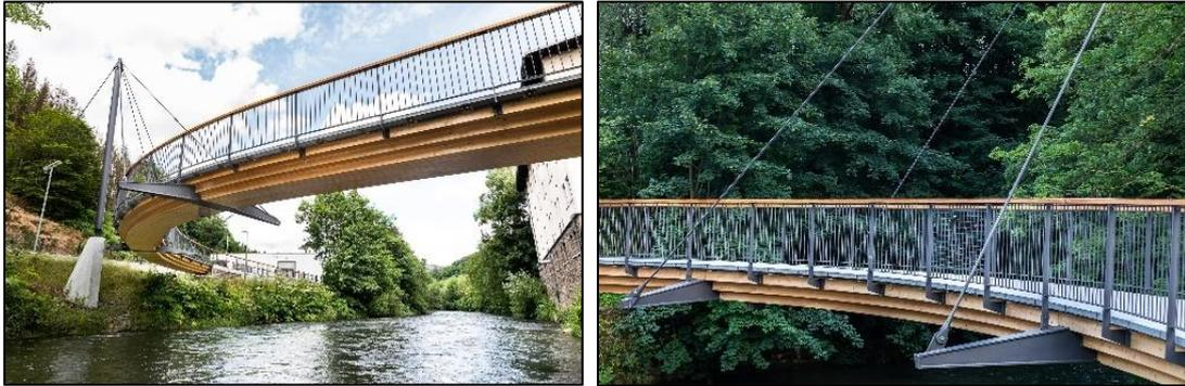
Figure 2. Photos of the intrados of the deck (left) and metallic connecting parts with the stay cables (right) [8]
