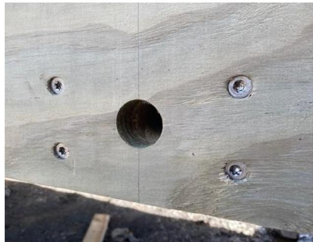
Photo 7: Fully threaded screws added behind the bearing plate to reduce pre-stressing losses.
