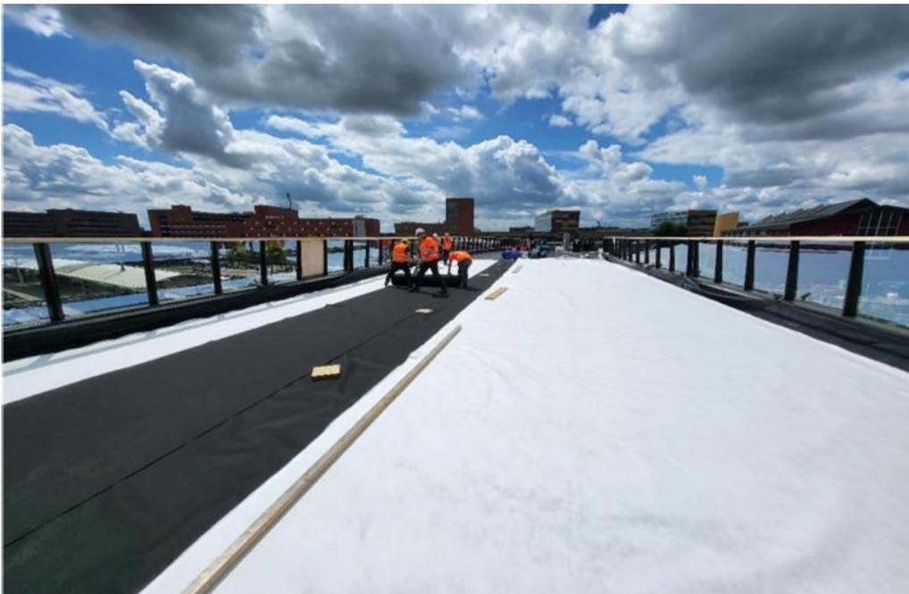
Figure 10: Installation of waterproofing with integrated full area leak monitoring
