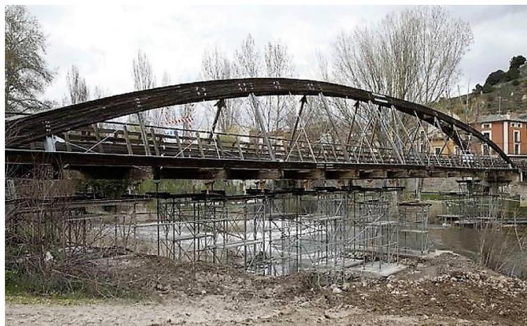
Figure 20: Shoring up the arches and deck, just before being dismantled.
