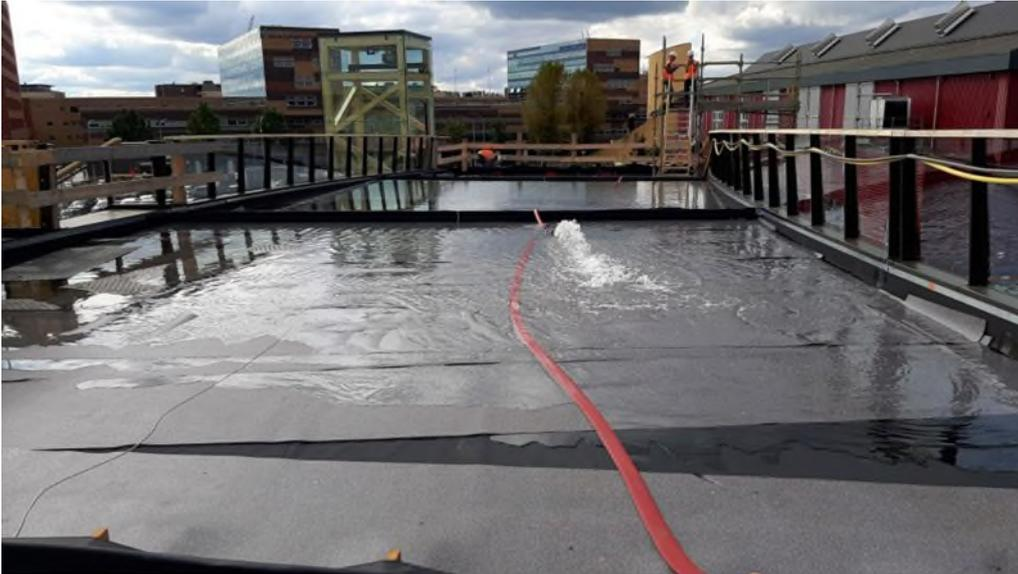
Figure 11: Flooded deck for integrity test
