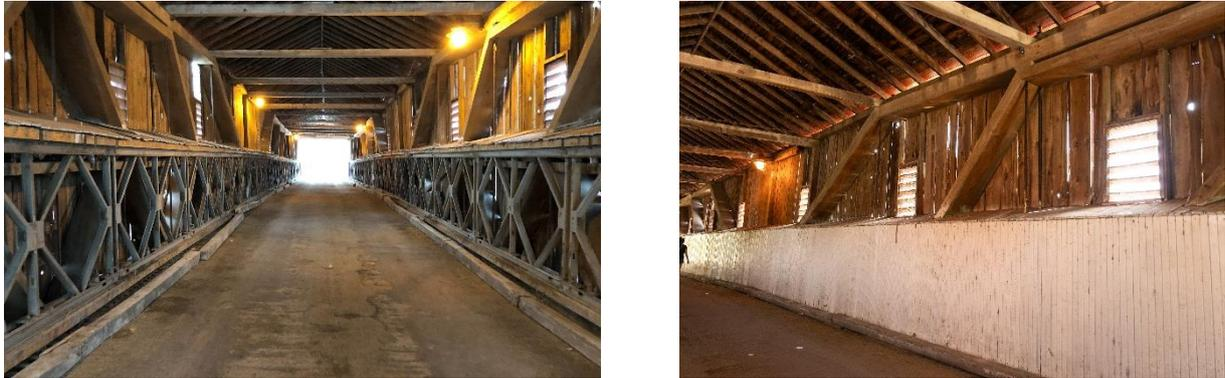
Figure 2. Steel Bailey trusses (left) and interior white wood cladding concealing steel trusses (right).
