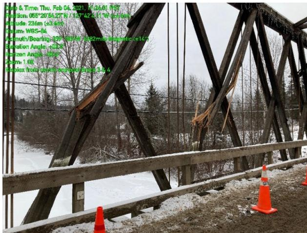
Figure 5. Badly Damaged Inner Diagonals
