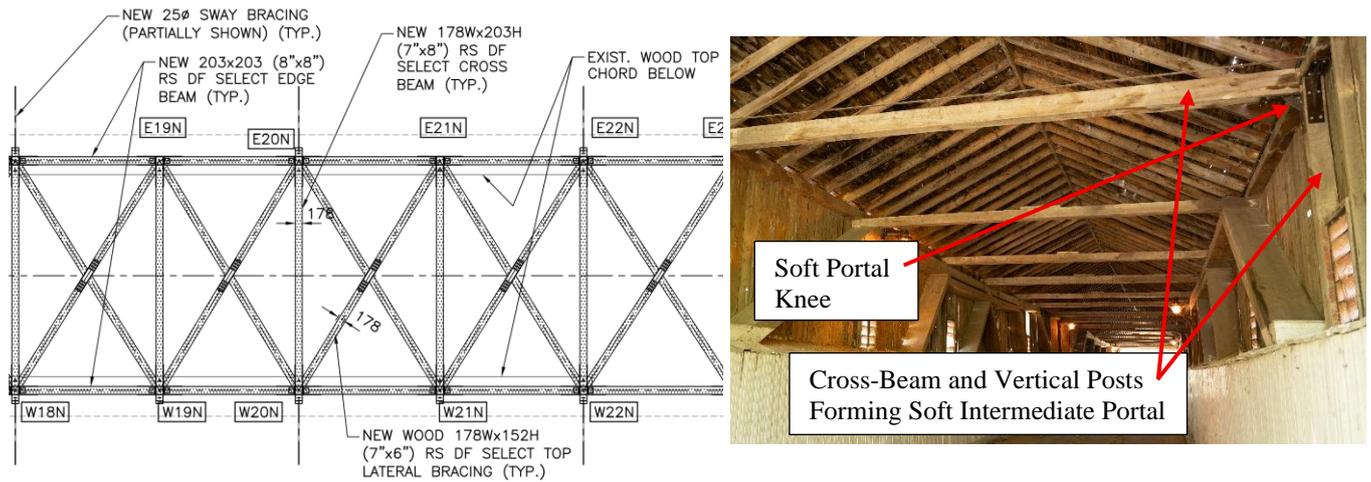
Figure 14. Excerpt of new wood top lateral bracing system (left) and intermediate portal frame in existing condition (right)
