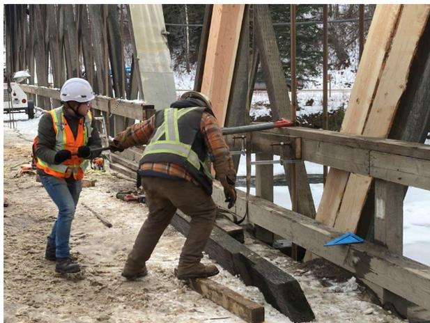
Figure 14 Re-tightening Tension Rod
