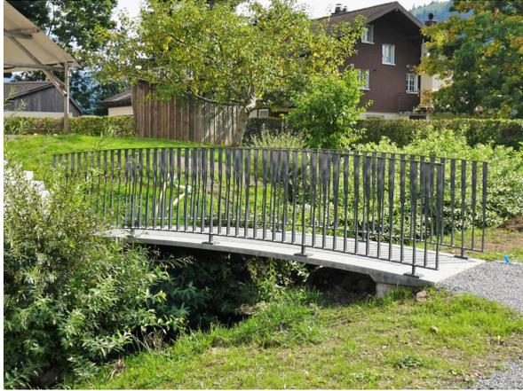
Figure 7: 4.5 m long and 6 cm thin UHPFRC bridge, Einsiedeln, Switzerland
