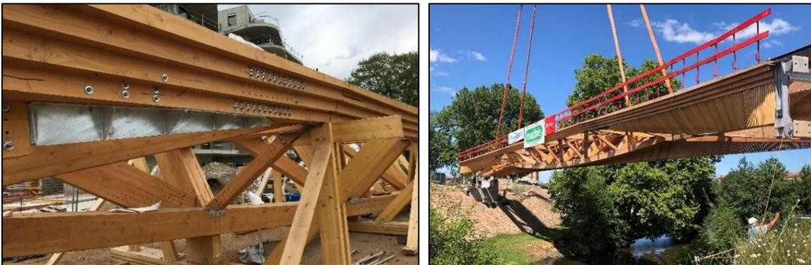
Figure 4. Photo of the structure being assembled (left) and during crane lifting (right) [10]
