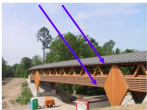
The angle of at least 30o to the vertical at which windblown rain is assumed to fall is shown in blue
