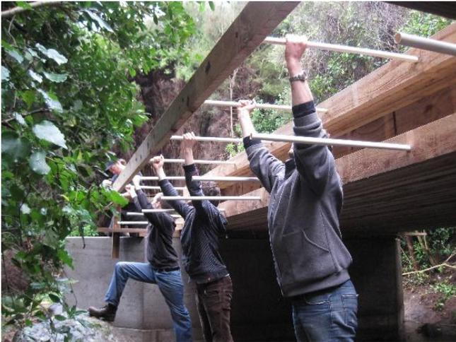
Figure 2. Boards being threaded one-by-one, over white plastic water pipes to locate and protect the tendons.
