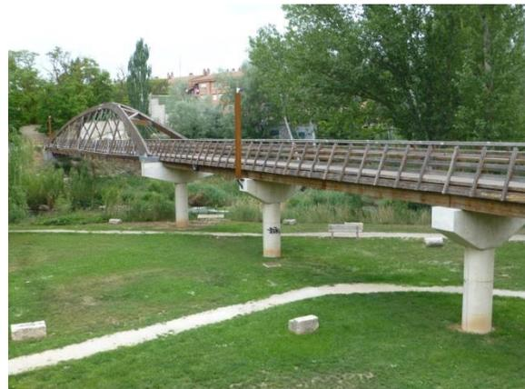
Figures 17, 18 and 19. New tie rods in August 2013, but distortions were really important in the month of May 2017.
