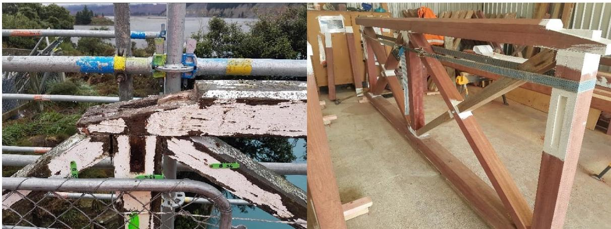
Figure 15. Numbering and deconstruction of balustrades.
