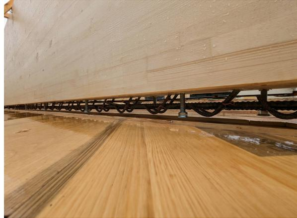
Figure 22: Detail of the pull- and shear connection
