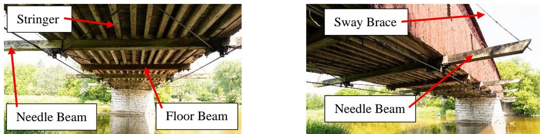
Figure 6. Typical floor system (left) and typical sway bracing at needle beam (right).
