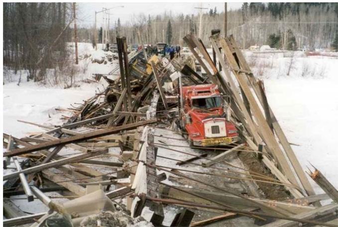
Figure 8. Willow Bridge Collapse After Vehicle Strike
