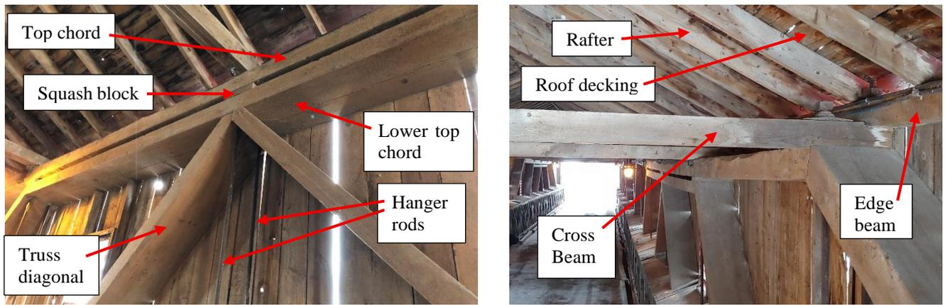
Figure 4. Wood truss members (left) and interior view of roof structure (right).
