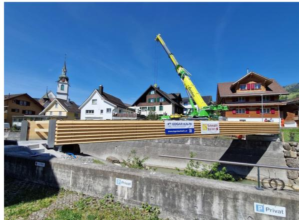
Figure 32: The bridge resting on the abutments; the temporary stabilisation of the timber beams is visible
