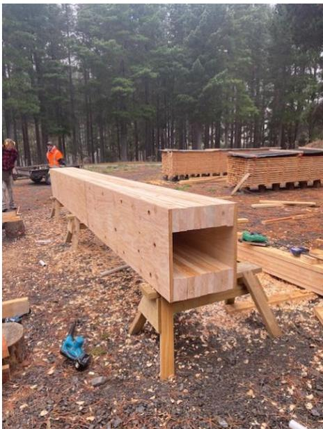
Photo 2: Pre-fabricated timber box girder module.
