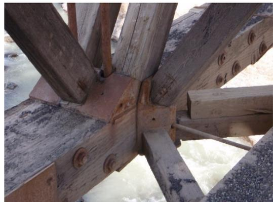
Figure 9. Typical Howe Truss Connection
