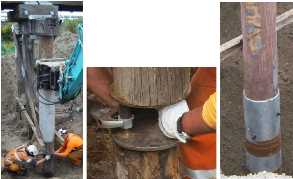
Figure 3: Current process for installing a stump repair.
