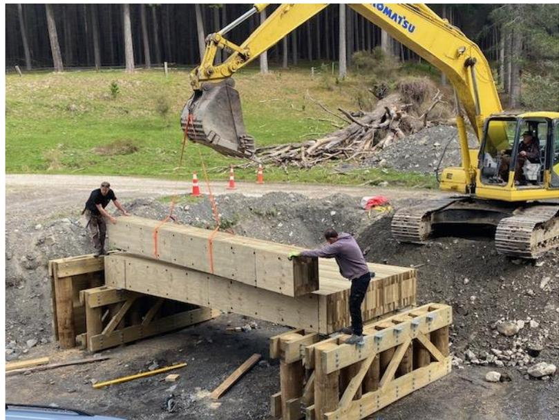
Photo 3. Assembly of the bridge deck/superstructure.
