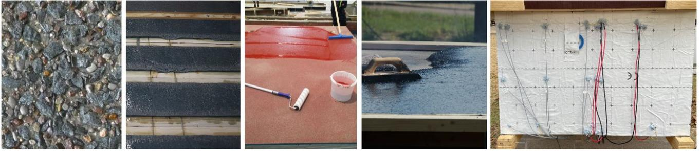
Figure 2. Fabrication of the superstructure segment; from the left to the right: Exposed aggregate surface; polymer mortar stripes; PMMA primer; pouring mastic asphalt; sealed end grain zone
