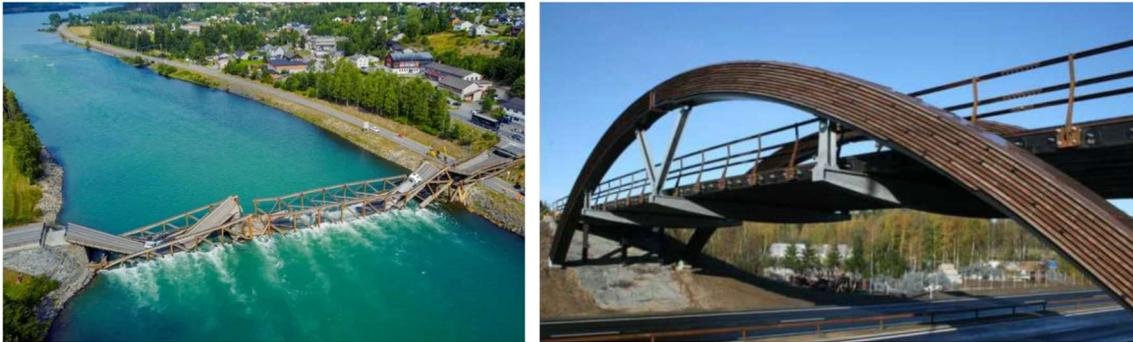
Figure 3. Tretten Bridge following the failure of a connection [1] (left) and Skogsrud Bridge with sacrificial fascia (right).
