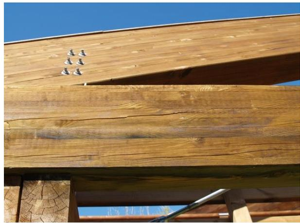
Figures 13 and 14. Deflections of the arches and cracks in the main beams.
