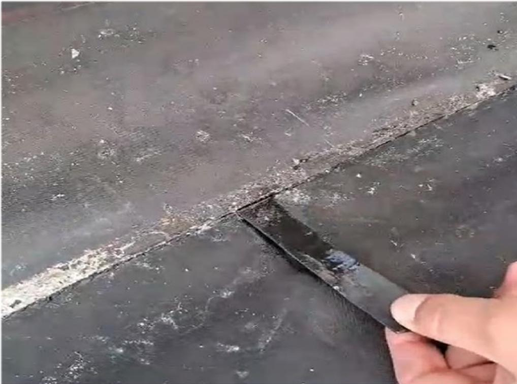
Figure 14: membrane leak identified and found with the installed full areal real-time monitoring system
