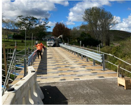
Figure 5 Engineered plywood panels soon after installation.
