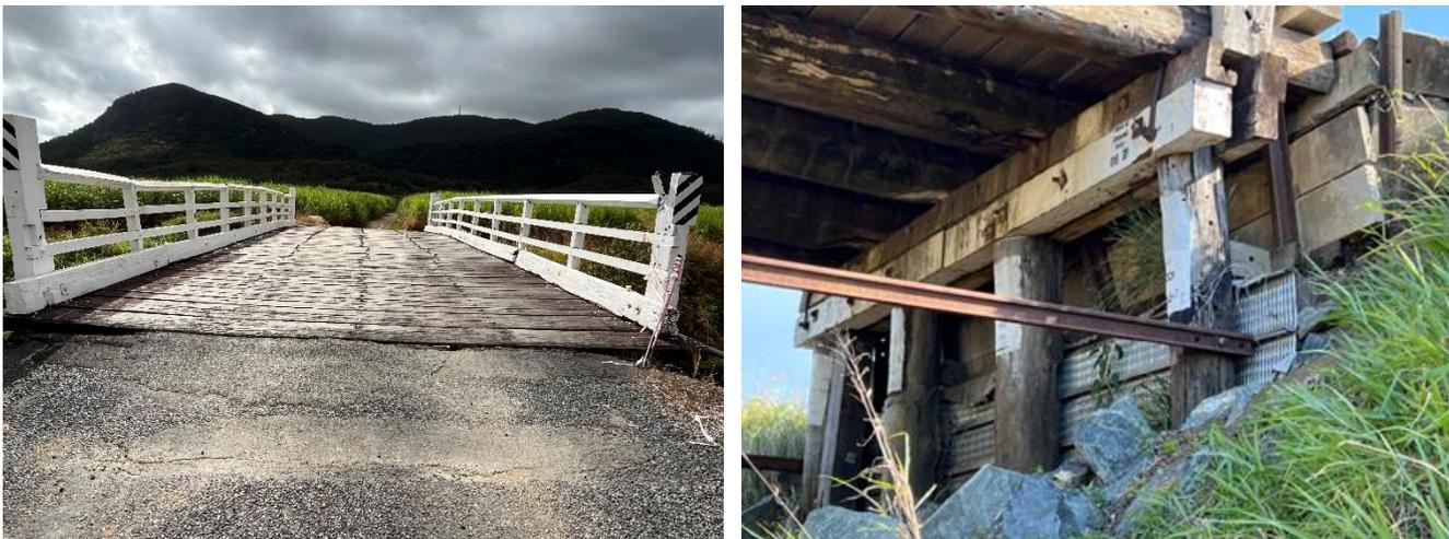
Figure 8. Approach settlement and abutment sheeting failure at Hopes Road Rail Overbridge
