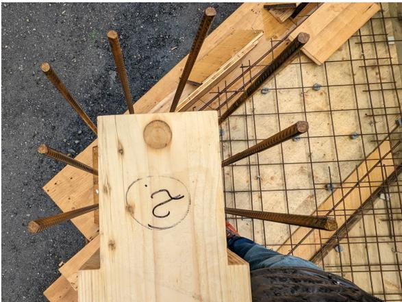
Figure 23: The reinforcement for the tilt protection
