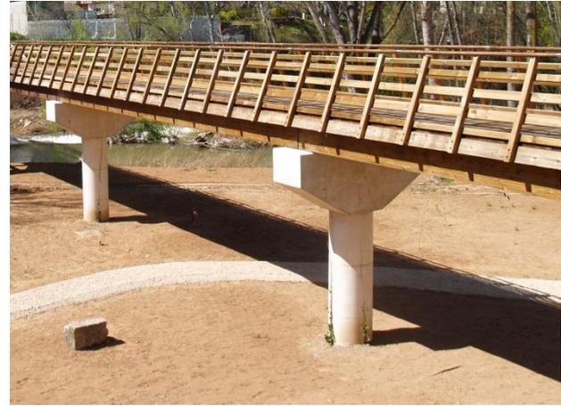
Figures 7 and 8. Both parts of the Peñafiel timber bridge.
