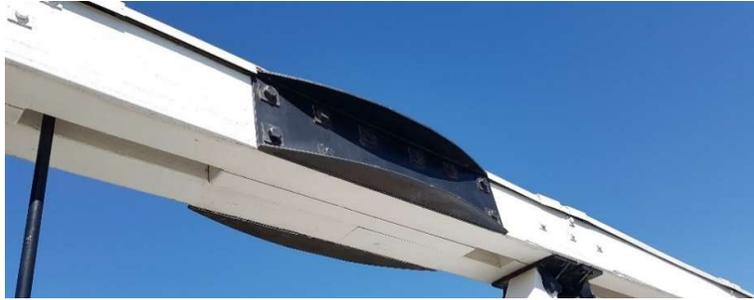
Figure 7. Flashing above top chord
