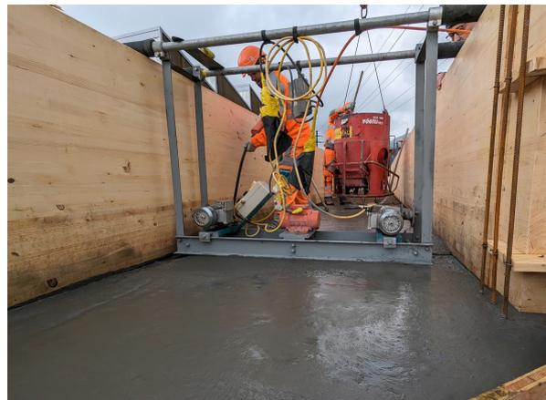
Figure 26: Smoothing the surface of the 1<sup>st</sup> layer
