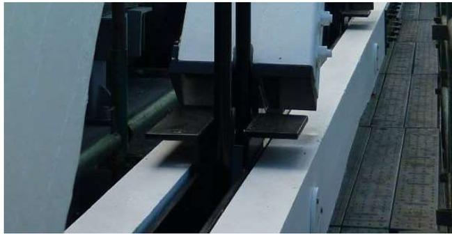
Figure 3. Pinned diagonal shoes connected at bottom chord steel plates
