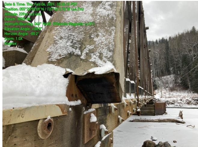
Figure 4. Dislodged End Diagonal (End Post)
