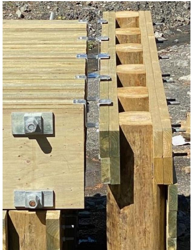
Photo 9: Bridge deck to abutment retaining wall detail, showing timber packing retention brackets.
