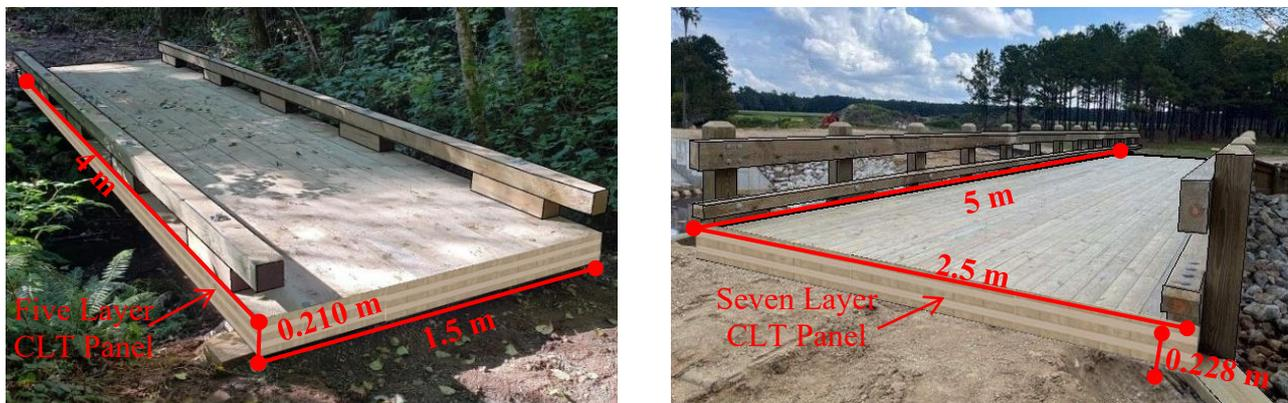
Figure 2. CLT panel application for short-span bridges.
