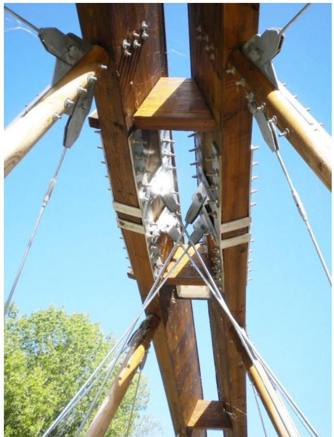
Figures 26, 27 and 28: Changes in the initial design of the bridge (left), and new rods (right)
