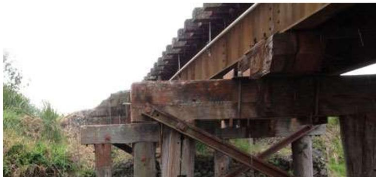
Figure 1. TePuke timber bridge exterior condition [10].
