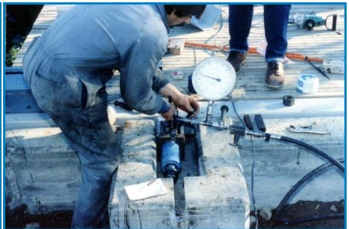
Figure 1(b). Post-tensioning in progress.
