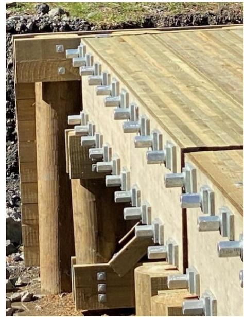
Photo 5: Stress laminated bridge deck.
