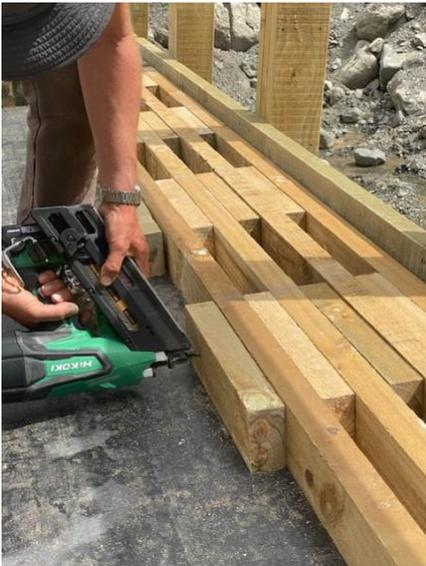
Photo 14: Nail lamination of timber lattice mat.
