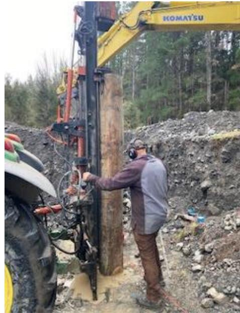
Photo 11: Tractor-mounted post driver used to drive timber piles for the support structure and the abutment retaining wall.
