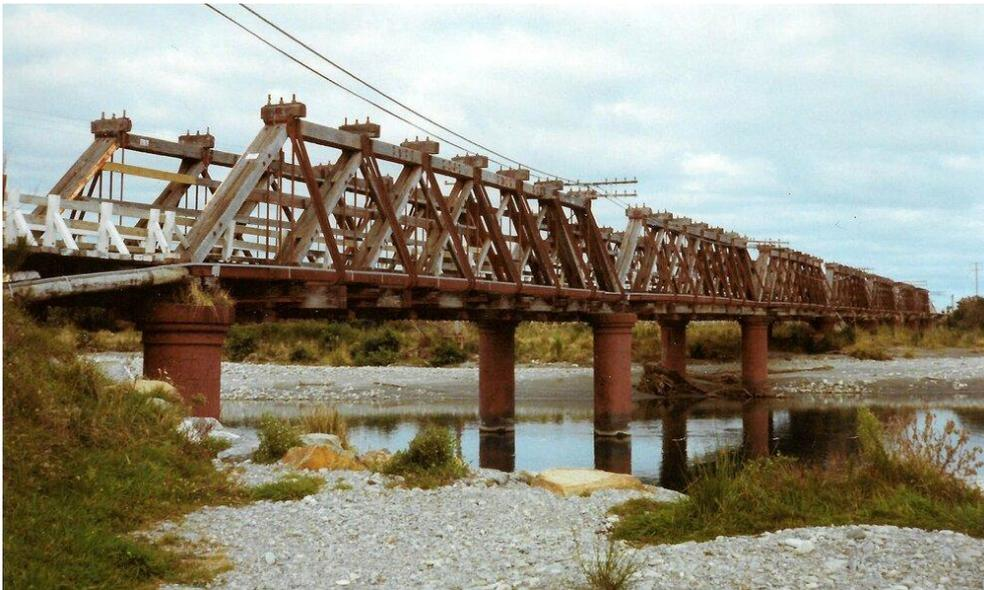
Figure 1 – A Howe-Truss bridge built from durable Australian hardwood typical of those which were common throughout the New Zealand road and rail networks in the first half of the 20<sup>th</sup> century.
