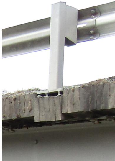
Figure 10 Local failure of laminated bridge deck under barrier impact
