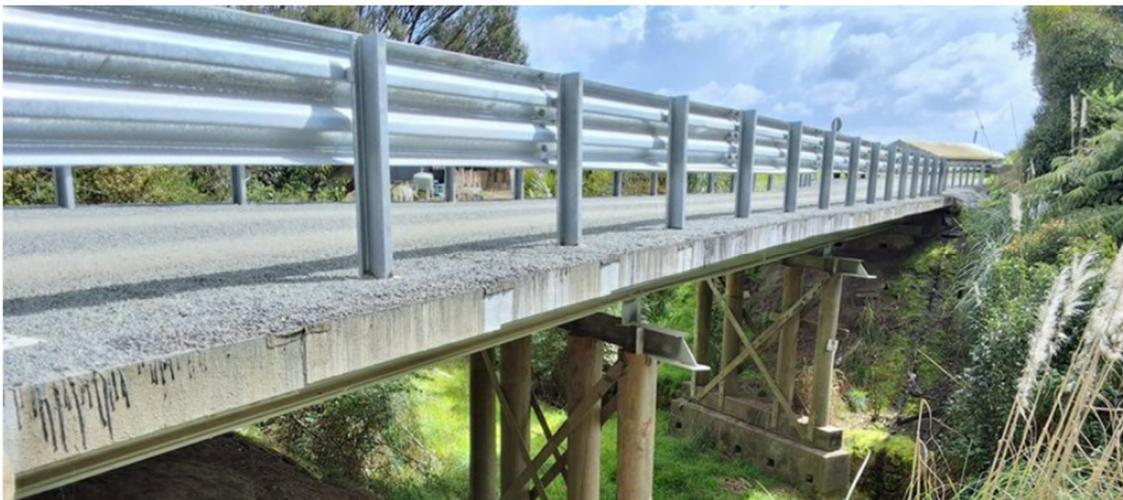
Figure 9 Chipseal extended to the edge of to prevent water pooling
