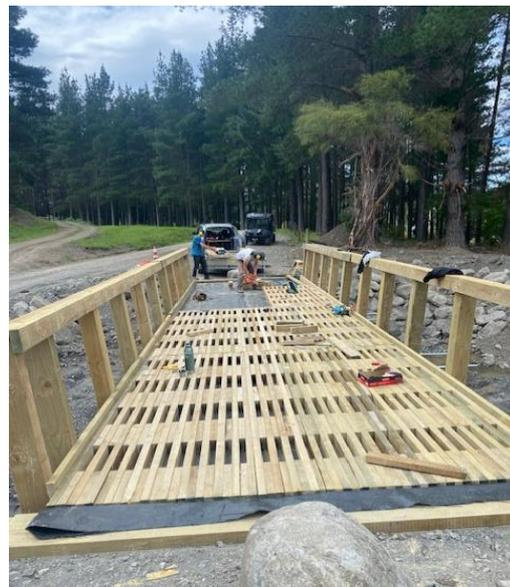
Photo 13: Timber lattice mat wearing course under construction.
