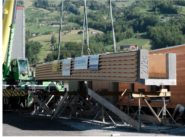
Figure 28: Lifting the bridge from the formwork
