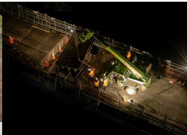
Figure 6. Installation of prefabricated deck sections during night closures.
