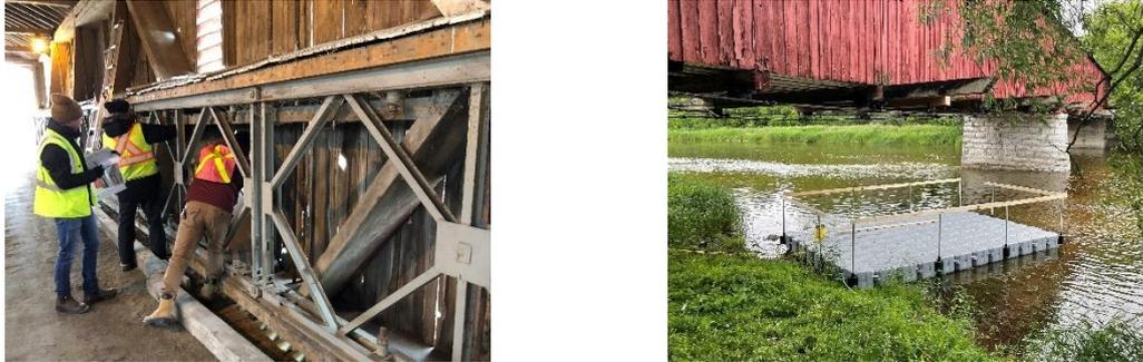
Figure 7. Wood truss inspection from deck level (left) and floating work platform for on-water inspection (right).
