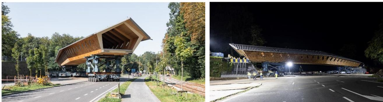
Figure 13. Transportation of the footbridge on SPMT from the prefabrication site to its final location ©Corentin Haubruge
