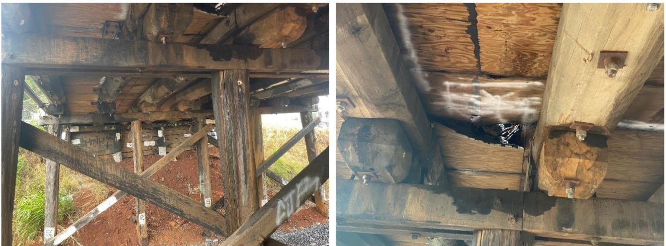
Figure 3. Rotten plywood deck sheeting at Drayton Rail Overbridge
