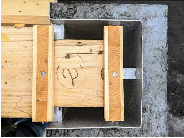
Figure 27: Detail of the tilt protection
