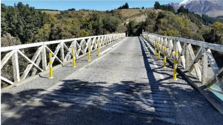
Figure 3. Poor deck condition (prior to replacement) and kerb delineation.
