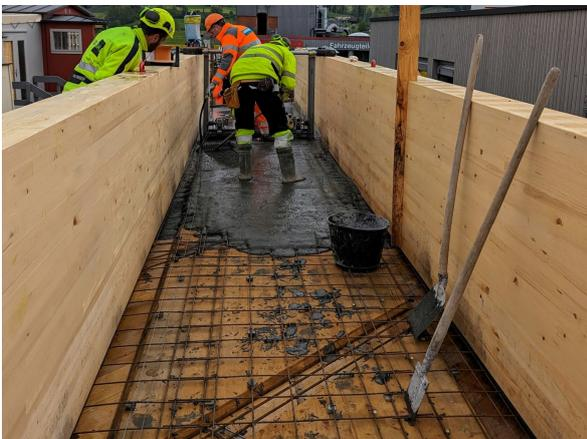
Figure 25: Casting of UHPFRC
