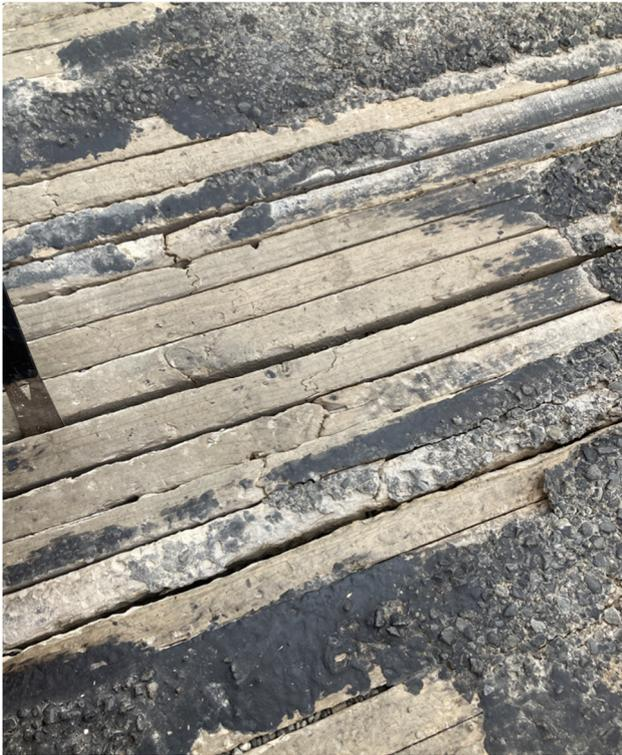
Figure 1 Delamination of surfacing on nail laminated bridge deck
