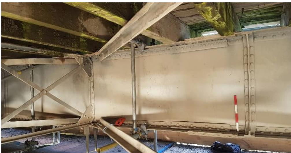
Figure 4. Original timber transoms notched to accommodate girder features.
