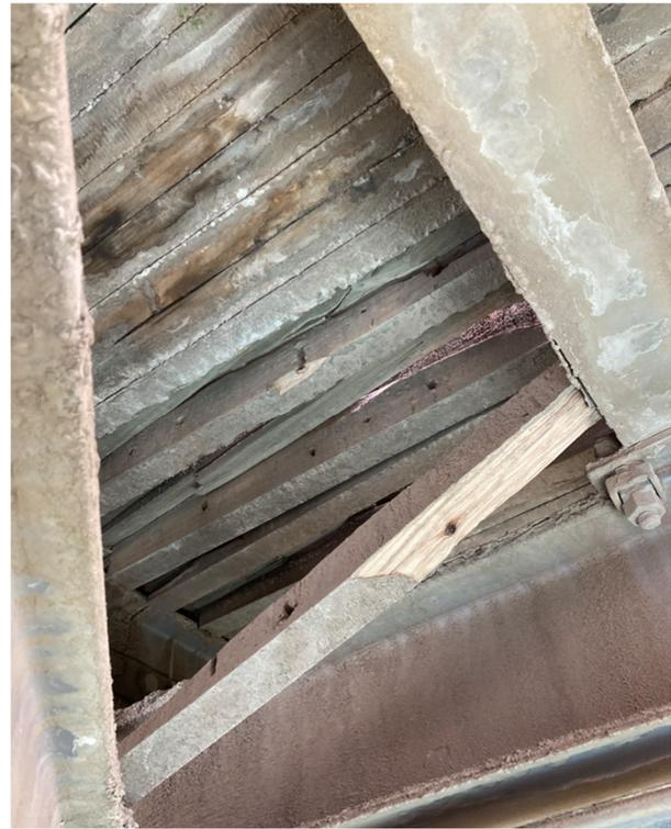
Figure 2 Failure of laminated bridge deck
