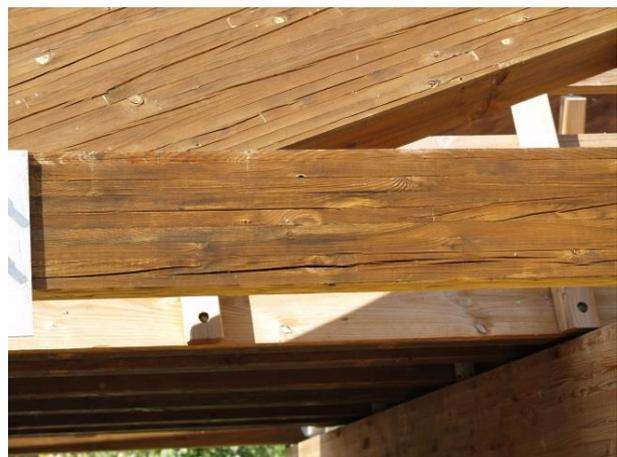
Figures 15 and 16: Delaminations in arches and beams.
