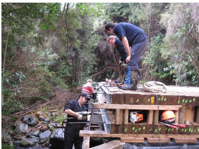
Figure 4. Post-tensioning in progress.
