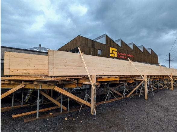
Figure 21: The timber beams on the formwork
