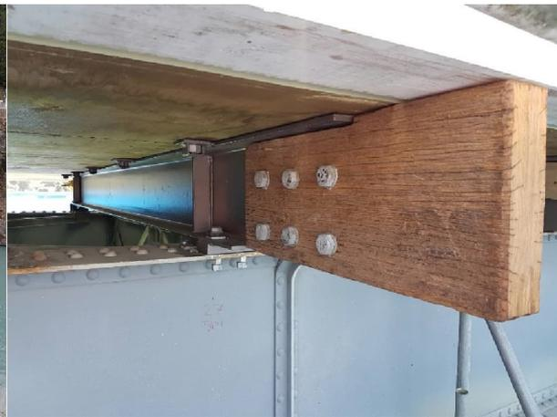
Figure 8. Spliced hardwood end piece (from original timber transom).
