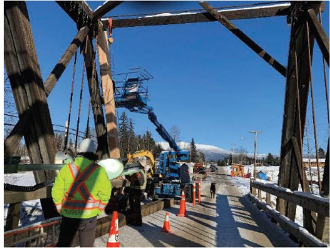
Figure 13 Replacement of Damaged End Post in Span 3
