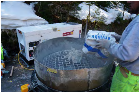
Figure 11: Rigiab bridge, Mixing UHPC
