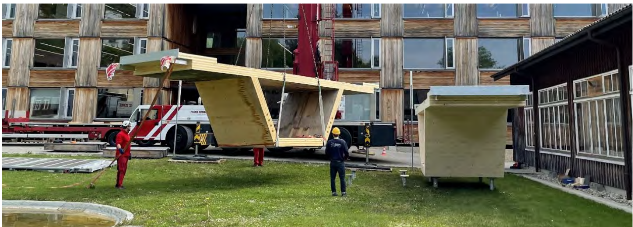
Figure 19: Installation of the box-girder modules. Picture: Steffen Franke
