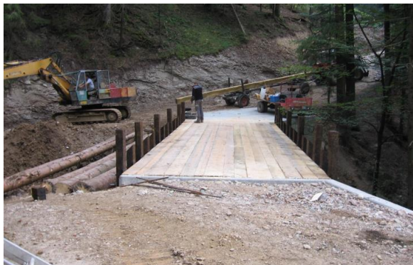
Figure 3: Modern interpretation of early log bridge by Prof Gehri. Untere Hürliisegg Bridge – Eggwil BE – constructed in 2009. This comes close to the historic "Schlagen einer Brücke", which refers to "Schlagen eines Baumes", in English cutting a tree/trunk with an axe. The wood was locally cut and processed on-site in order to arrange it as a bridge (deck) for forest-traffic. Pictures: E. Gehri
