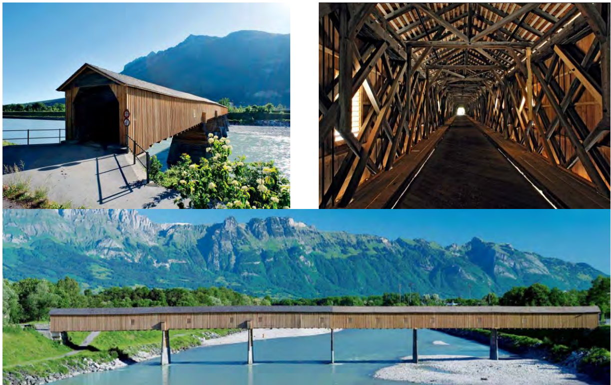
Figure 11: Howe truss bridge crossing the river Rhine between Sevelen (CH) and Vaduz (LI). Built (opened) in 1871/1901 it was one of a series of more than 10 Howe truss bridges along the river Rhine, including one for railway. It is the only one that still exists. This bridge was under road-traffic load (6t) until in 1975 a new pre-stressed concrete bridge (from which the picture at the bottom was taken) was built next to it. www.swiss-timber-bridges.ch/ lists a total of 34 Howe truss bridges that exist(ed) in Switzerland. Pictures: Documentation: Die alte Rheinbrücke Vaduz–Sevelen
