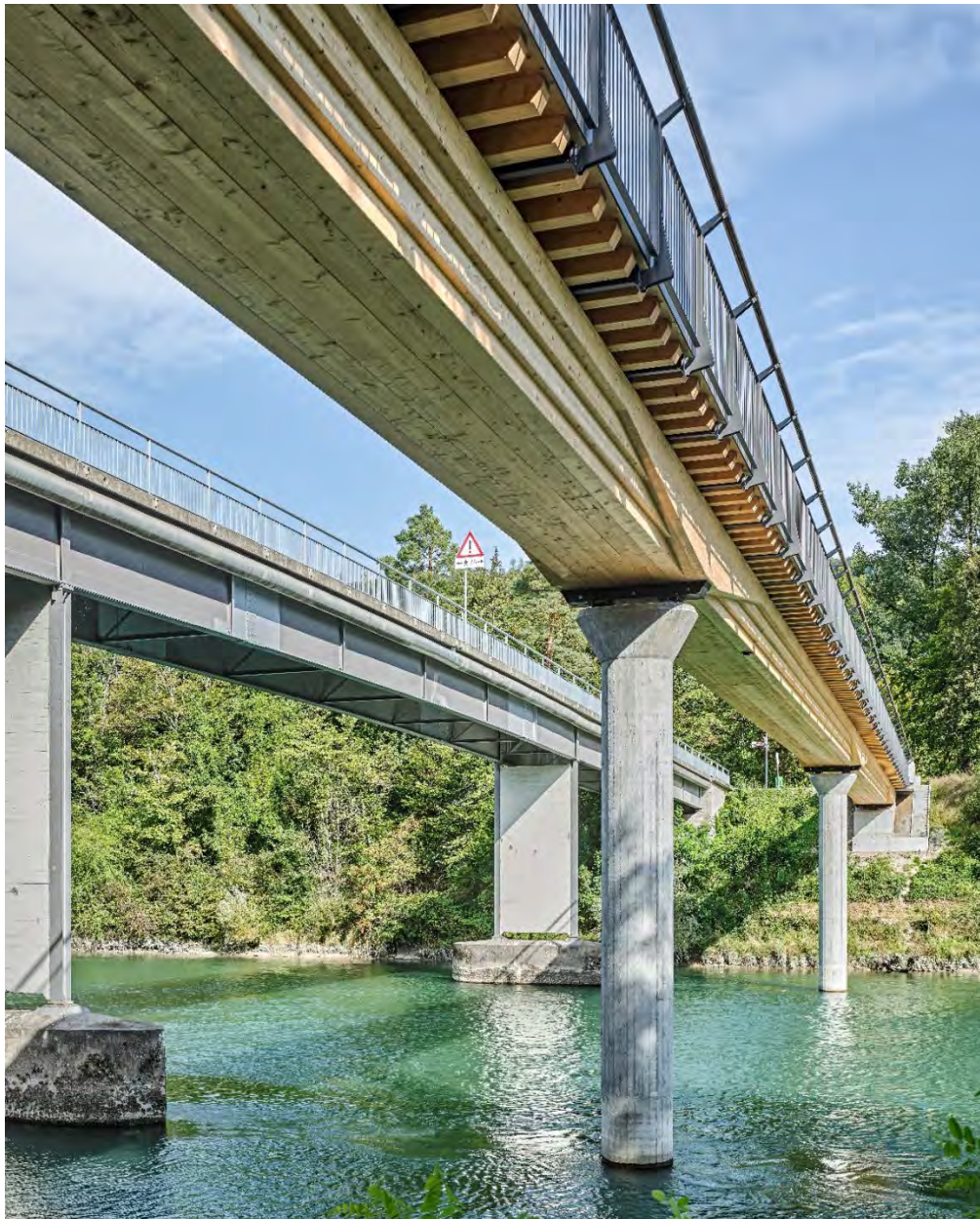
Figure 1: Bridge B, three-span girder next to the existing road bridge [Roger Frei, Zurich]
