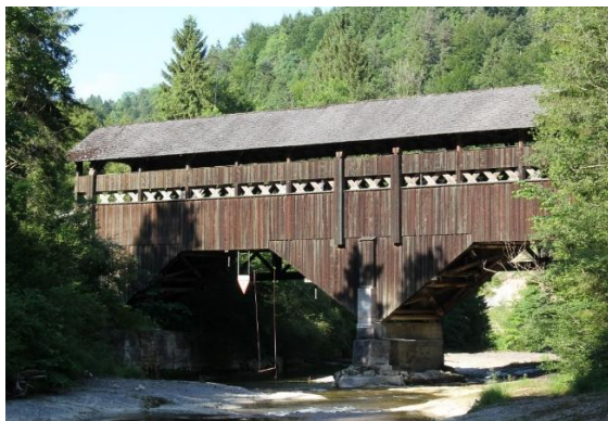
Figure 10: Necker Bridge Anzenwil SG from 1863 with it's main structural elements being Town lattice trusses. The bridge spans 46 meters (with the addition of an intermediate support) and was under road traffic load until the year 2000, when a modern concrete-steel hybrid bridge was set next to it. The new bridge carries the main traffic load and leaves the slow traffic to the old timber bridge, Pictures: R. Widmann
