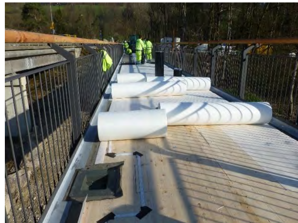
Figure 14: Sensors on the wooden panel and laying of the glass fleece and PBD seal
