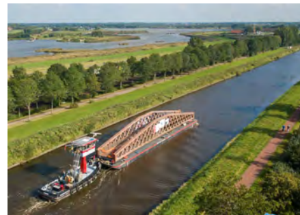
Figure 5: Aerial photo of the 'Pieter Smitbrug' along with a detail of the main span (above) and the main span and transport for the production site in Kampen to the building location by boat.
