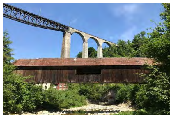
Figure 2: Timber, iron and stones (masonry). Kubel-bridge (1776) with a span of 30 m in the first plane and Sitterviadukt (1910) with a length of 365 m and a maximum span of 120 m. With 99 m this is the highest railway bridge in Switzerland. Picture: R. Widmann
