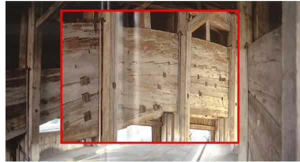
Figure 9: Another Emme bridge (in Schüpbach) with an impressive 49 m span and similar construction as Hasle-Rüeggsau and Wettingen bridges. The picture shows nicely the technics used to create an arch with interlocking tooth-shaped recesses in the lamellae and/or hardwood dowels for the transfer of shear forces within the arch. Picture: E. Honegger (A. Steurer) [6]
