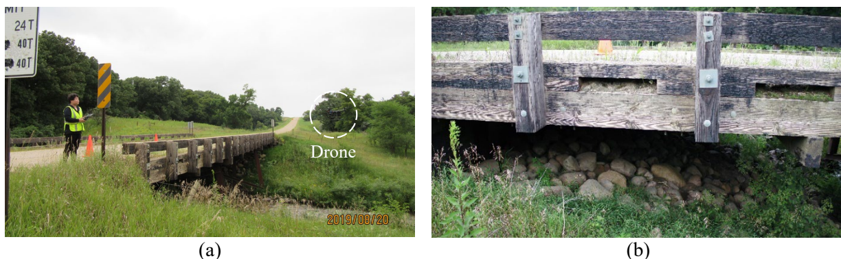
Figure 1: Bridge inspection: (a) drone-aided bridge inspection and (b) inspection images captured by DJI Matrice 210.
