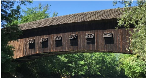
Figure 8: Bridge at Hasle-Rüeggsau BE crossing the river Emme. Built in 1839, it has a span of 58 m and thus is very similar to the Grubenmann Bridge in Wettingen, Picture: R. Widmann
