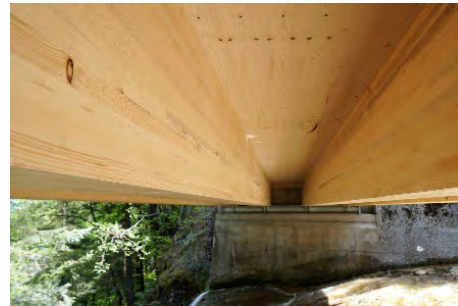
Figure 22: Fruttli bridge, soffit with beams and 3-layer panels
