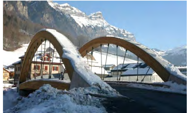
Figure 27: Kirchenbrücke Muotathal, Canton Schwyz built 2009, Lenght: 34,00 m Span: 33,40 m, 40 tons, arch bridge, Design: Pirmin Jung, Rain, BPP Ingenieure, Schwyz, E. Imhof, Luzern, Picture: BFH
