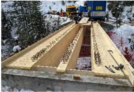
Figure 9: Rigiab bridge, the glulam girders placed on the abutments
