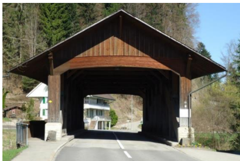
Figure 14: Dörfli-Bridge, Eggiwil, Canton Bern, built 1985, Span 30.6 m, Live load 28 Tons, Type Covered arch bridge, Design: H. Vogel and Prof. Gehri, ETH Zürich, Pictures: Archiv K. Schwaner.
