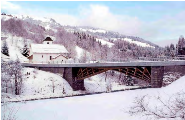
Figure 20: Glenner-bridge, Graubünden, built 2002, Length 34,6 m, / Span 24,6 m, Live load 4x75 Tons, Design: Conzett, Bronzini, Gartmann AG, Chur, Pictures: Graubündenh Holz, Landquart/LIGNUM
