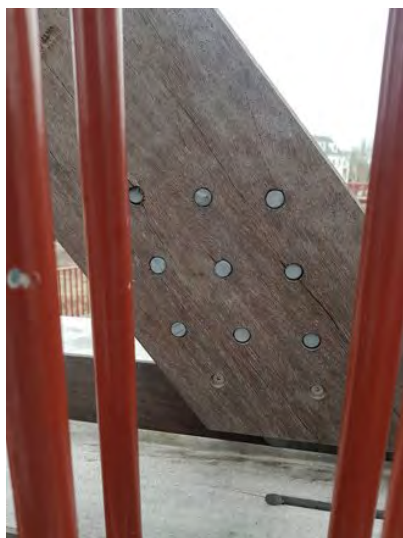
Figure 2 dowelled connection
