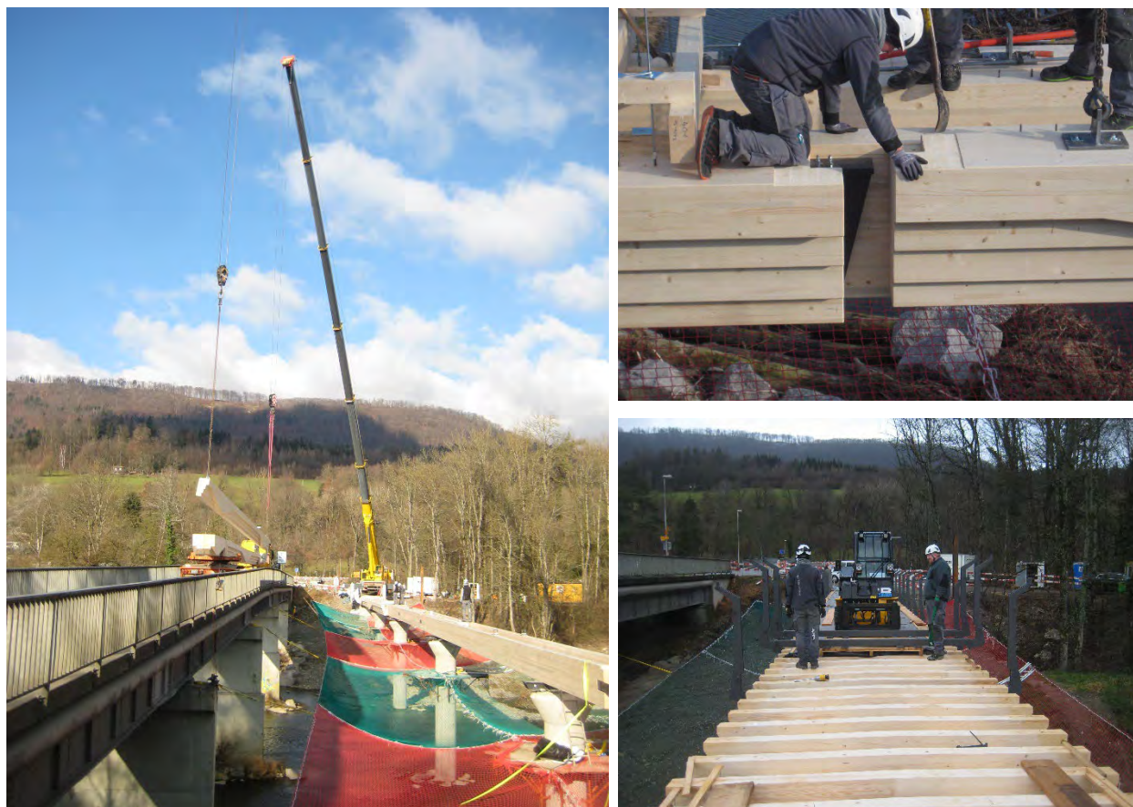
Figure 6: left: pendulum lift; above: connection of the main girders; below: installation of crossbeams and railing frames
