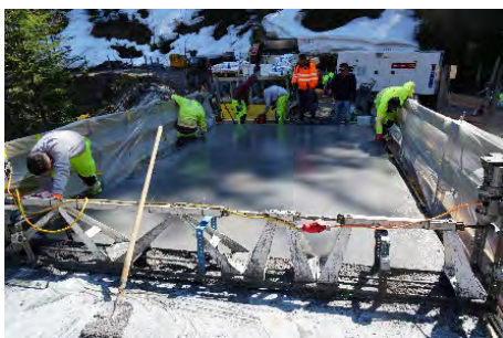
Figure 15: Rigiab bridge, smoothing of the first layer of the UHPC deck
