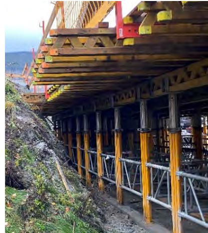
Figure 11 Våla bru – scaffolding on flood-plain (photo: H. E. Wedum)
