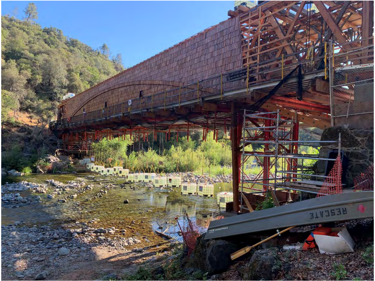
Figure 6 – Load testing bridge prior to shoring removal (Lawrence Jones)
