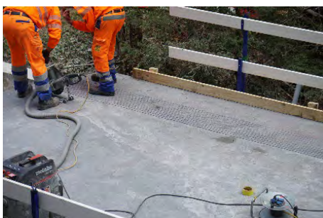
Figure 17: Fruttli bridge, Milling the grooves to increase skid resistance
