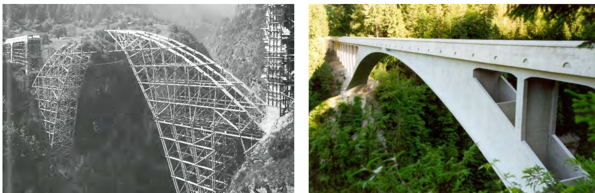
Figure 12: Renowned Salginatobelbrücke in Schiers, Graubünden, Eastern Switzerland by Robert Maillard (concrete structure) and Richard Coray (timber scaffolding) 1929-1930. These pictures highlight the transition of the role of timber in bridge constructions from being the dominant permanent solution in the past to serving as a temporary auxiliary construction. Pictures: L. Gianadda, R. Widmann
