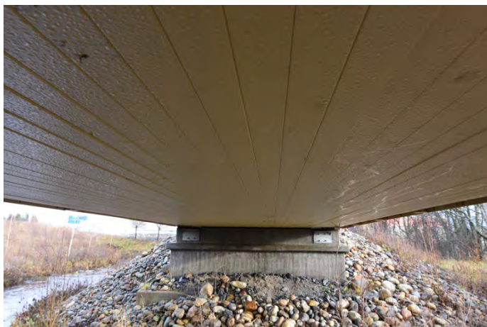
Figure 2. Condensation on bottom of the bridge deck.
