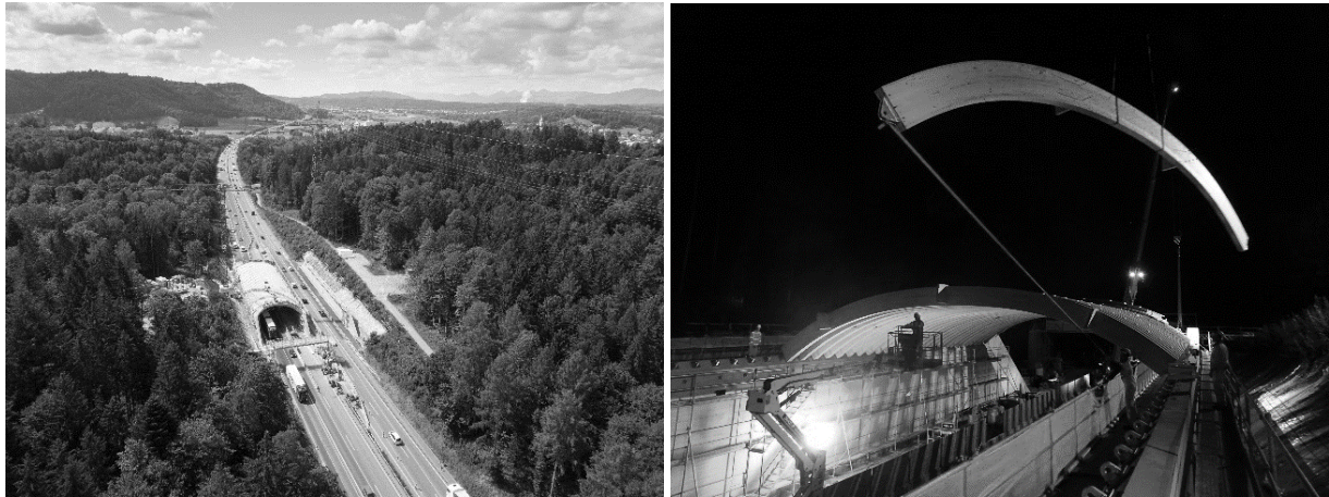
Figure 8 Assembly of the individual trusses between the portal modules.
