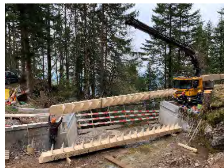
Figure 8: Fruttli bridge, Assembly of the girders with the pre-assembled formwork
