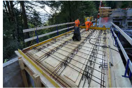
Figure 10: Fruttli bridge, the reinforced bridge slab
