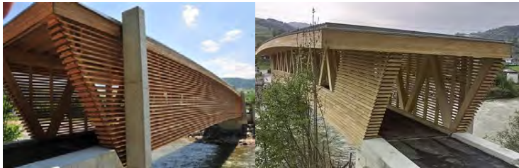
Figure 26: Luthernbrücke, Canton Luzern built 2010, Lenght: 13,55 Span: 13.05 m, 40 tons, block glued girder bridge, Design: E. Winkler & Partner, Luzern, Makiol + Wiederkehr, Beinwil, Picture: Makiol + Wiederkehr
