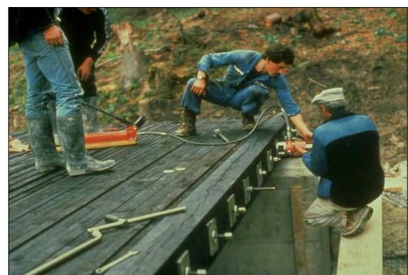
Figure 17: Forestry-Bridge-Typ with Stress Laminated Timber Deck Plates, Design: Prof. E. Gehri, Pictures: Archiv K. Schwaner.
