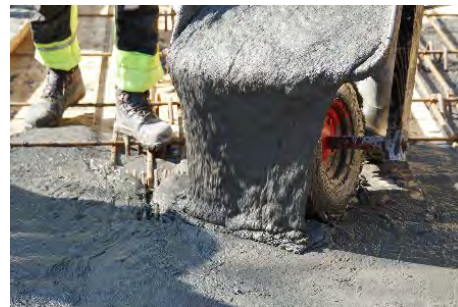
Figure 14: Rigiab bridge, casting of the UHPC
