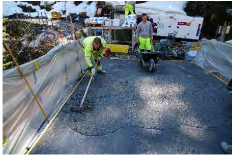
Figure 19: Rigiaa bridge, casting the second layer
