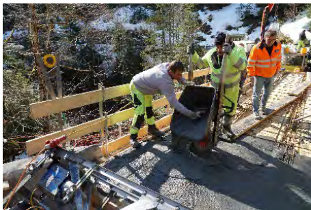
Figure 13: Rigiab bridge, casting of the UHPC
