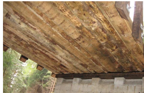
Figure 3: Modern interpretation of early log bridge by Prof Gehri. Untere Hürliisegg Bridge – Eggwil BE – constructed in 2009. This comes close to the historic "Schlagen einer Brücke", which refers to "Schlagen eines Baumes", in English cutting a tree/trunk with an axe. The wood was locally cut and processed on-site in order to arrange it as a bridge (deck) for forest-traffic. Pictures: E. Gehri
