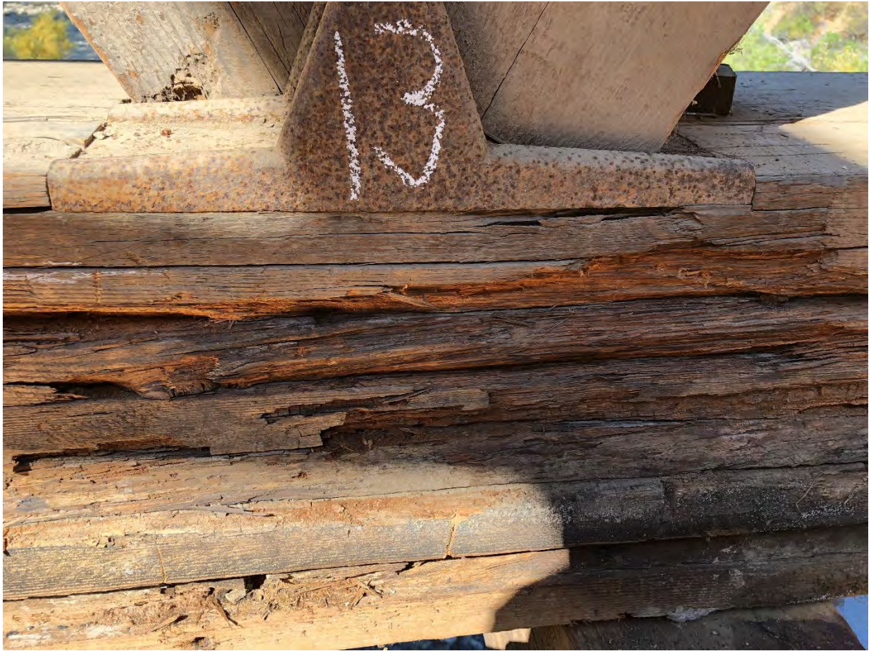
Figure 3 – Photograph of Bottom Chord Decay prior to repair (Lawrence Jones)
