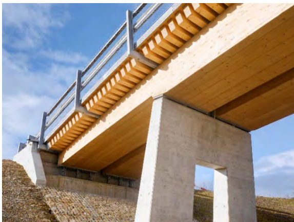
Figure 1: Bridge Horen Switzerland, block glued glulam members as main structural elements, Source: BFH, Switzerland
