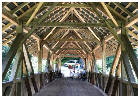
Figure 5: Letzibrücke from 1853 crossing the river Necker in Canton Thurgau. This is an example for a composite truss frame. Since 1969 a pre-tensioned concrete bridge close to the timber bridge takes the road traffic. The picture on the right shows how historic timber bridges can be used in Switzerland nowadays. Like many others they can be, e.g. rented for events like weddings or birthdays. This possibility of use contributes to the fact that the local population often has a strong emotional bond with "their" wooden bridge and thus also takes care of the structure. Pictures: R. Widmann
