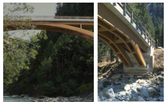
Figure 23: Crestawaldbrücke in Sufers, Graubünden, Timber-Concrete-Composite, built 1996; Span 31 m; 28 tons, Engineers W. Zöllig, Arbon, M. Krattiger, Happerswil, Pictures: Archiv K. Schwaner
