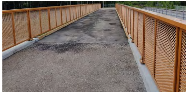
Figure 3: The bridge during and after construction. Left: Stage 1 with only the timber structure. The vertical flat bars for the railings were present on the bridge. Right: Finished bridge (stage 3 and 4) with timber structure, railings and asphalt.
