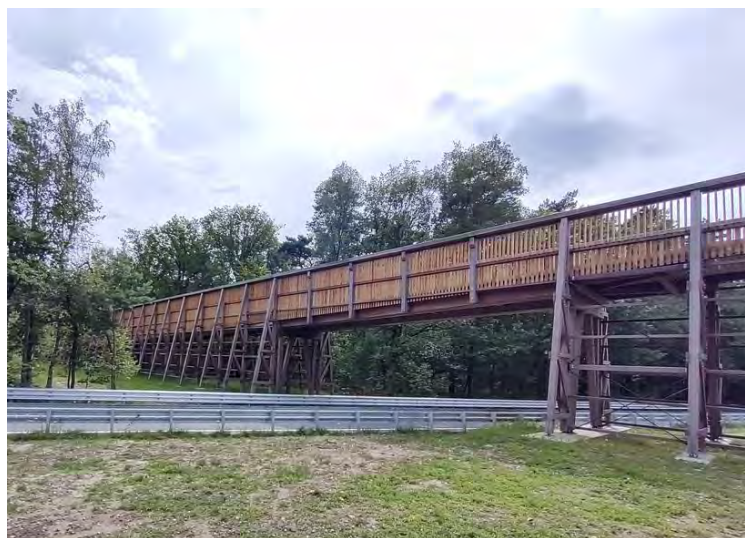
Figure 3: 15 meter span of the 'Fietsen door de Heide' with dowel laminated beams
