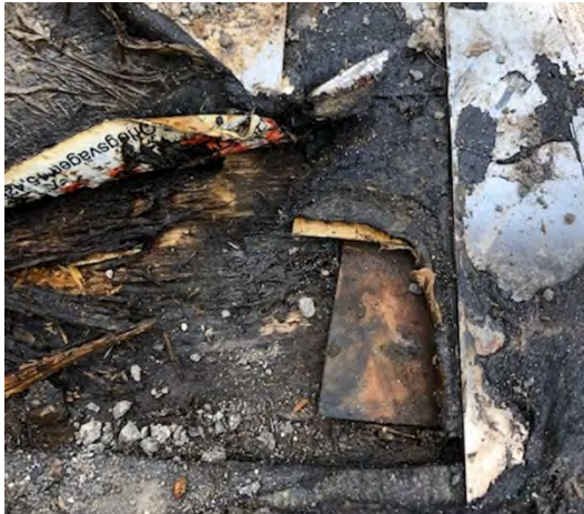
Figure 6. Detail of Gislaved bridge. Membrane strip not properly attached. Decayed wood is also visible.
