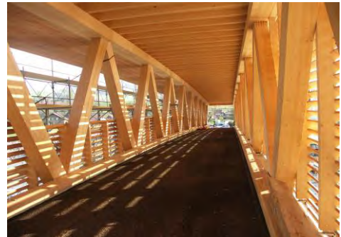
Figure 28: Enningerbrücke, Malers, Canton Luzern, built 2010, Lenght: 46,0 m Span: 42,0 m, 28 tons, truss bridge, Design: Pirmin Jung, Rain, Emch + Berger WSB AG, Luzern, Pictures: Kolb, Pirmin Jung Ingenieure
