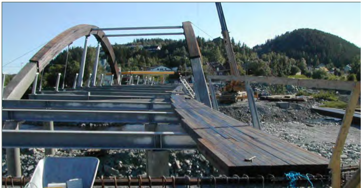
Figure 2: Stress laminated deck of sawn timber on steel cross beams (Måsørbrua)
