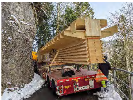
Figure 7: Rigiaa bridge, Transport of the girders with pre-assembled formwork
