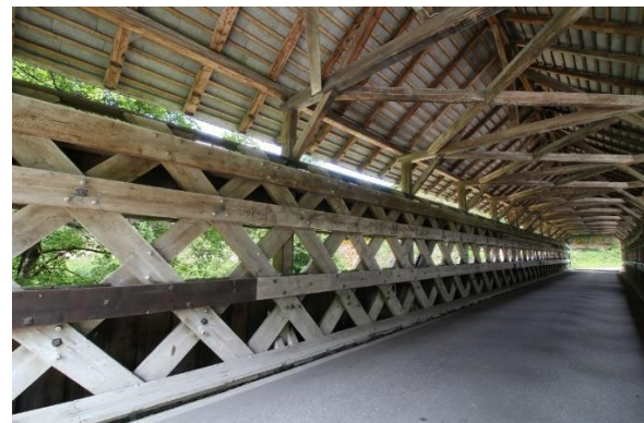
Figure 10: Necker Bridge Anzenwil SG from 1863 with it's main structural elements being Town lattice trusses. The bridge spans 46 meters (with the addition of an intermediate support) and was under road traffic load until the year 2000, when a modern concrete-steel hybrid bridge was set next to it. The new bridge carries the main traffic load and leaves the slow traffic to the old timber bridge, Pictures: R. Widmann
