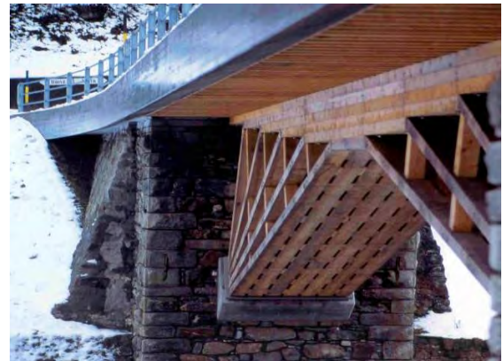
Figure 20: Glenner-bridge, Graubünden, built 2002, Length 34,6 m, / Span 24,6 m, Live load 4x75 Tons, Design: Conzett, Bronzini, Gartmann AG, Chur, Pictures: Graubündenh Holz, Landquart/LIGNUM
