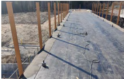
Figure 3: The bridge during and after construction. Left: Stage 1 with only the timber structure. The vertical flat bars for the railings were present on the bridge. Right: Finished bridge (stage 3 and 4) with timber structure, railings and asphalt.
