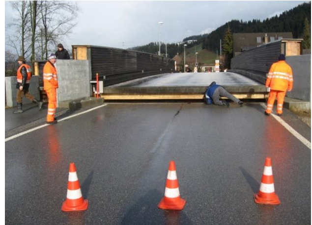
Figure 24: Obermattbrücke, Canton Bern, built 2007, Through Bridge, vertically adjustable (70 cm) bridge when high water, span: 32 m live load 40 tons, Design: Paul Grunder AG, Täufen, Pictures: BFH
