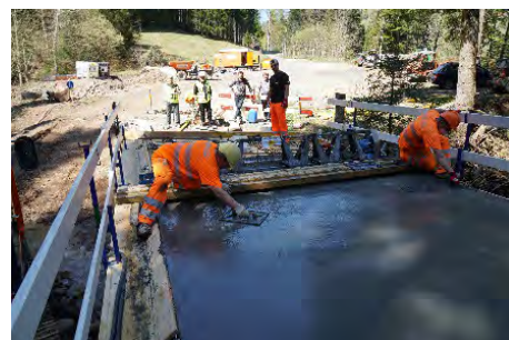
Figure 16: Fruttli bridge, smoothing of the UHPC deck
