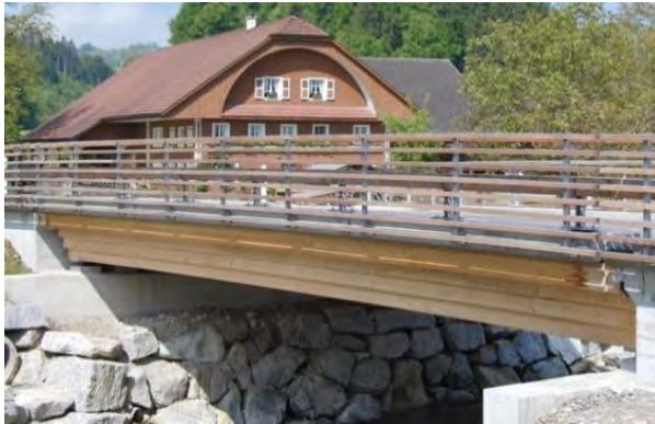
Figure 26: Luthernbrücke, Canton Luzern built 2010, Lenght: 13,55 Span: 13.05 m, 40 tons, block glued girder bridge, Design: E. Winkler & Partner, Luzern, Makiol + Wiederkehr, Beinwil, Picture: Makiol + Wiederkehr
