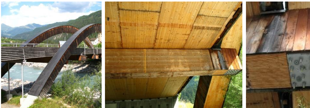
Figure 19: Bridge San Nicla, Canton Graubünden, built 1993, Length/Span: 47,8/39 m, Live load 28 Tons, Type Arch Bridge, Design: A. Mayer, Sent, A. Deplazes, Chur, Prof. E. Gehri, Pictures: BFH
