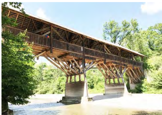
Figure 5: Letzibrücke from 1853 crossing the river Necker in Canton Thurgau. This is an example for a composite truss frame. Since 1969 a pre-tensioned concrete bridge close to the timber bridge takes the road traffic. The picture on the right shows how historic timber bridges can be used in Switzerland nowadays. Like many others they can be, e.g. rented for events like weddings or birthdays. This possibility of use contributes to the fact that the local population often has a strong emotional bond with "their" wooden bridge and thus also takes care of the structure. Pictures: R. Widmann
