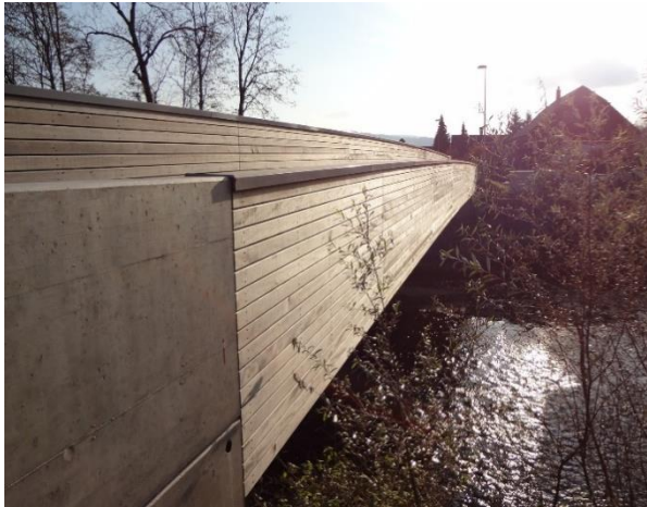
Figure 24: Obermattbrücke, Canton Bern, built 2007, Through Bridge, vertically adjustable (70 cm) bridge when high water, span: 32 m live load 40 tons, Design: Paul Grunder AG, Täufen, Pictures: BFH
