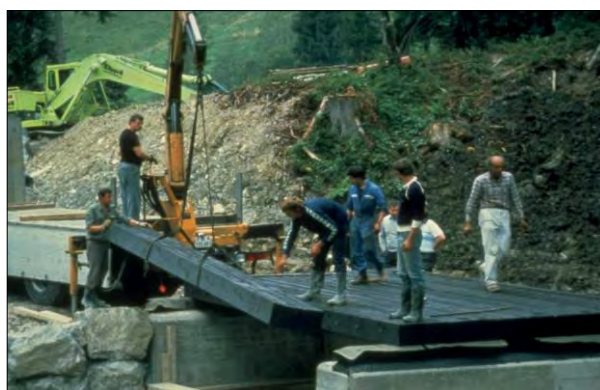
Figure 17: Forestry-Bridge-Typ with Stress Laminated Timber Deck Plates, Design: Prof. E. Gehri, Pictures: Archiv K. Schwaner.
