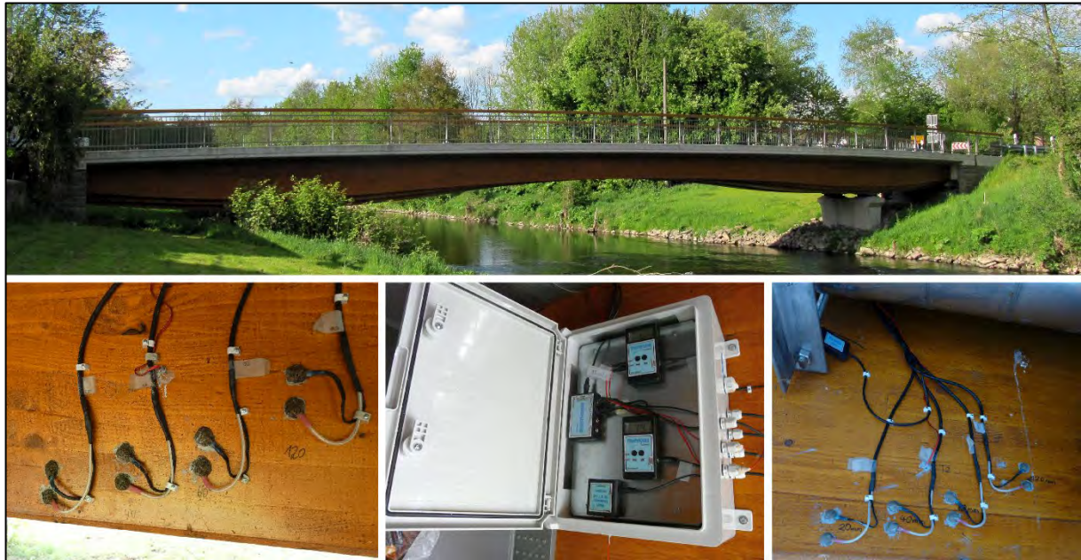
Figure 2: View of the TCC road bridge in Lohmar-Schiffarth (top of the image); measuring area over the foreland (bottom left); measuring equipment in an installation box (bottom centre); measuring area over the River Agger (bottom right of the image)
