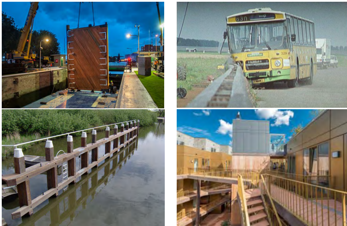
Figure 1: several examples of the use of ekki in timber structures other than bridges (from left to right, high to low): Lock gates (Bernhardsluis, Deventer), guide rail (during tests, Lelystad), fenders (location unknown), and stairways and balconies (Kop van Lombok, Utrecht)
