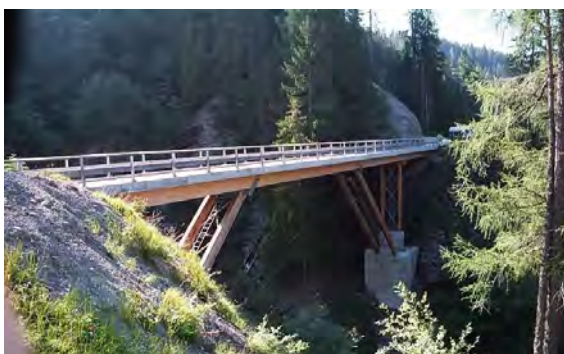
Figure 22: Ronatobelbrücke in Furna, Graubünden, Timber-Concrete-Composite, built 1991; Span 12-12-13,75-12,25 m; 28 tons, Engineers Buchli + Joh. Fromm, Picture: Andrea Bernasconi HES-SO Yverdon/LIGNUM
