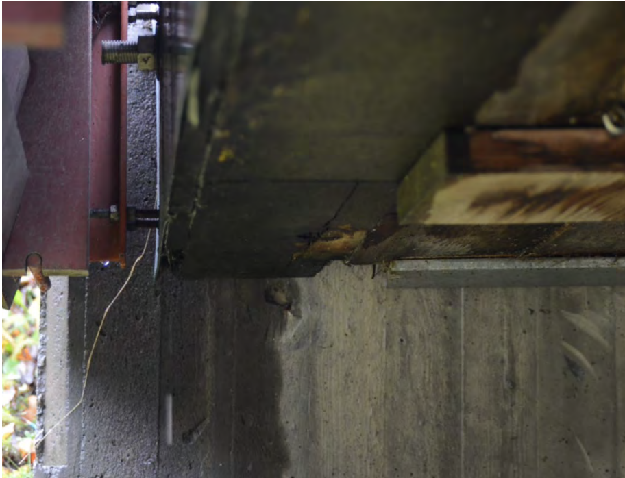
Figure 1. Wet outer beam from Klockarleden short.
