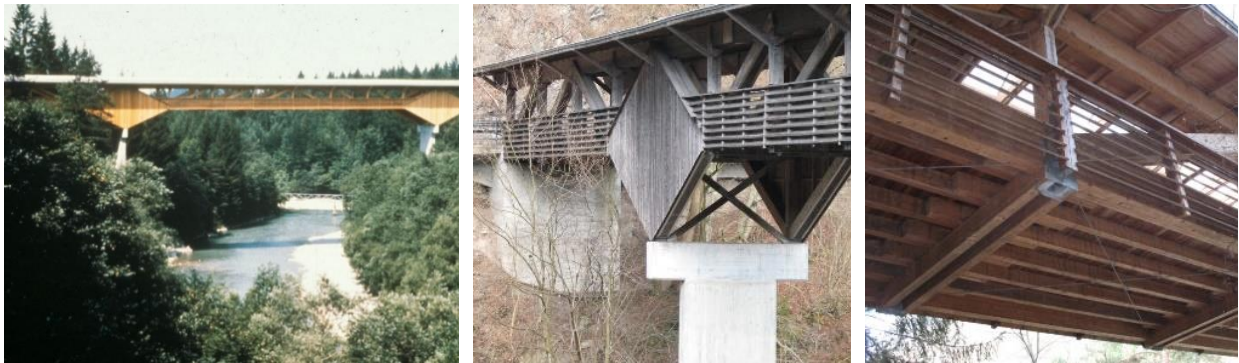
Figure 18: Cycle Path Bridge over Simme near Reutigen/Wimmis, Canton Bern, built 1989, Length 108 m, /Span 27/54/27 m, Type Covered truss bridge, Design: J. Natterer, Pictures: Kolb. Schwaner.
